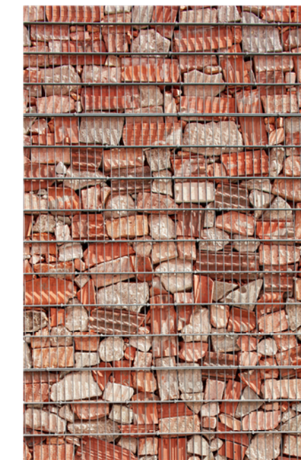
Gabion Wall (mix of site-recycled red brick and stone)
