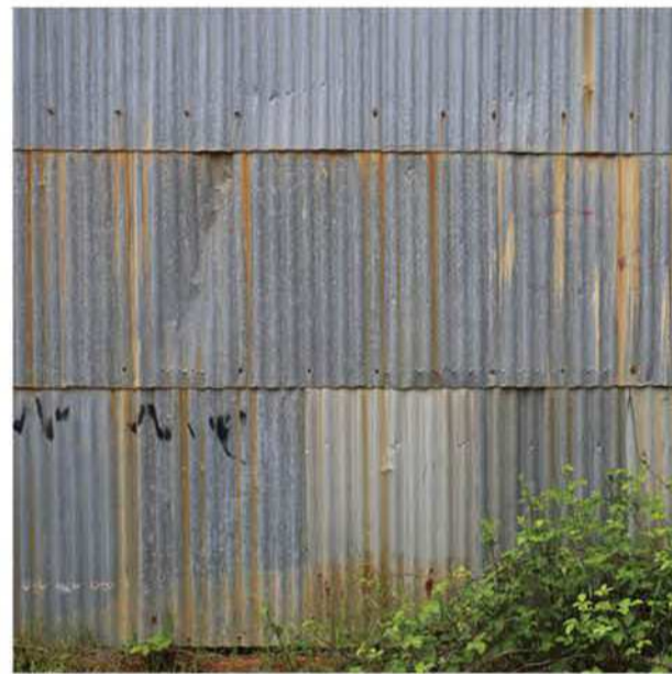
4 REUSED CORRUGATED METAL SHEETING * EXTERNAL CORRUGATED METAL CLADDING TO ALL MACHINE BAYS TO BE REMOVED AND STORED TO ALLOW FOR INSTALLATION OF NEW RAINSCREEN ON THE OUTSIDE OF THE EXISTING STEEL STRUCTURE - ONCE RAINSCREEN IS INSTALLED THE EXISTING CLADDING WILL BE REUSED TO PROVIDE CONSISTENT LOOK TO ALL MACHINERY SHEDS
