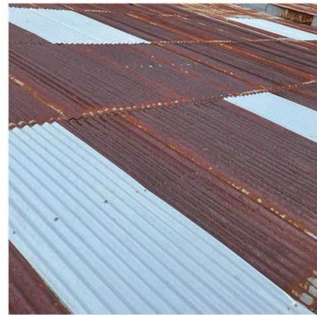
4 REUSED CORRUGATED METAL SHEETING * EXTERNAL CORRUGATED METAL CLADDING TO ALL MACHINE BAYS TO BE REMOVED AND STORED TO ALLOW FOR INSTALLATION OF NEW RAINSCREEN ON THE OUTSIDE OF THE EXISTING STEEL STRUCTURE - ONCE RAINSCREEN IS INSTALLED THE EXISTING CLADDING WILL BE REUSED TO PROVIDE CONSISTENT LOOK TO ALL MACHINERY SHEDS
