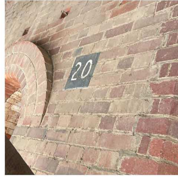
1 EXISTING MASONRY * UNDERTAKE A "LIGHT CLEAN" OF BRICK SURFACES TO REMOVE DUST, DIRT, ANY "NON-HERITAGE" GRAFFITI, AND ANY HANGING RESIDUE ON CEILING UNLESS INDICATED DIFFERENTLY. * DISCOLORATION AND TRACES OF THE FIRING PROCESS ARE TO BE LEFT INTACT WHERE IT IS POSSIBLE TO DO SO.
