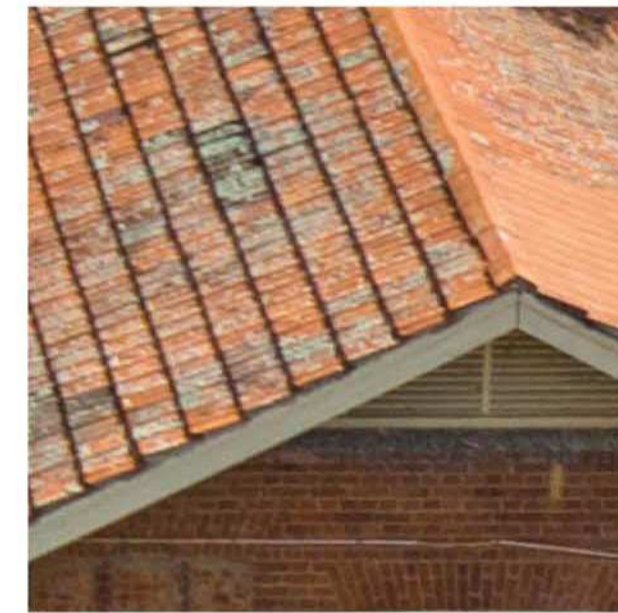
12 CERAMIC ROOF TILES (EXISTING REUSED)
