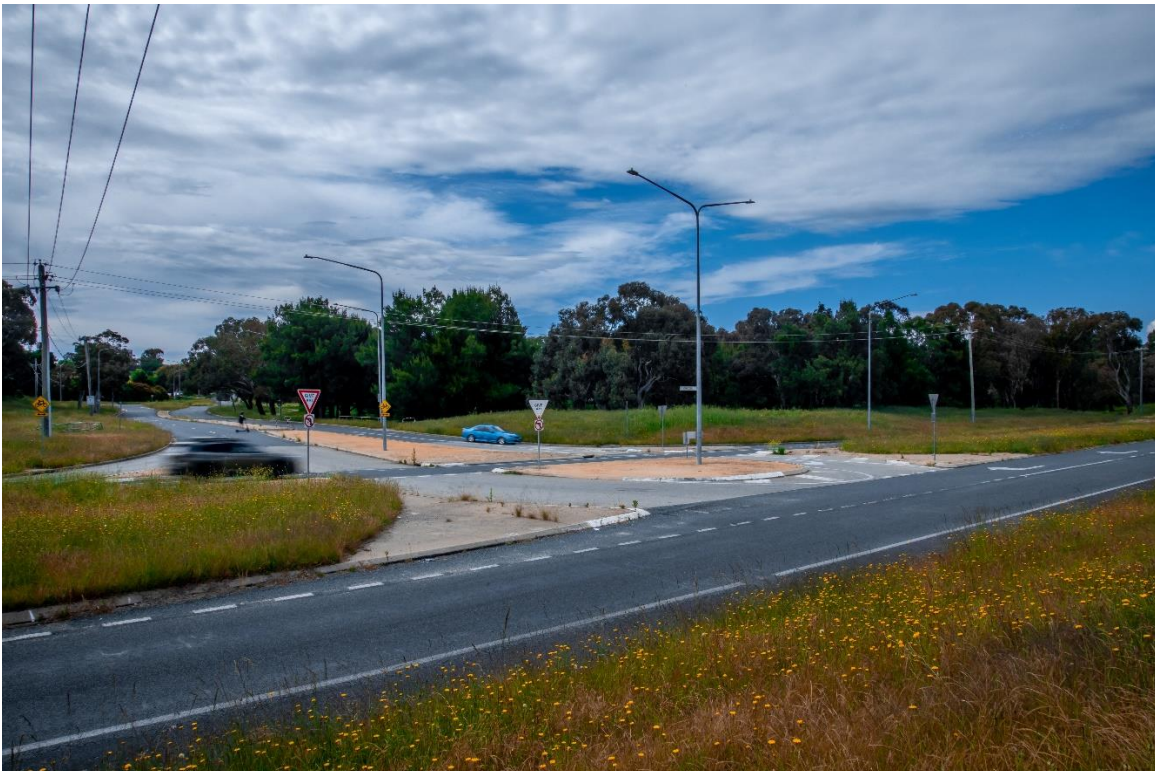
Figure 2-2 | View facing southeast of the Athllon Drive and Fincham Cres intersection, existing condition
