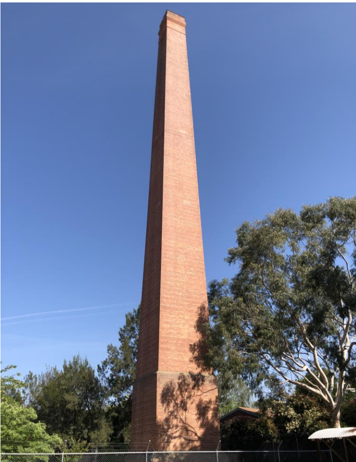
Photo 17.2 Chimney Stack for Hardy Patent Kiln 2 (Umwelt, 2020)
