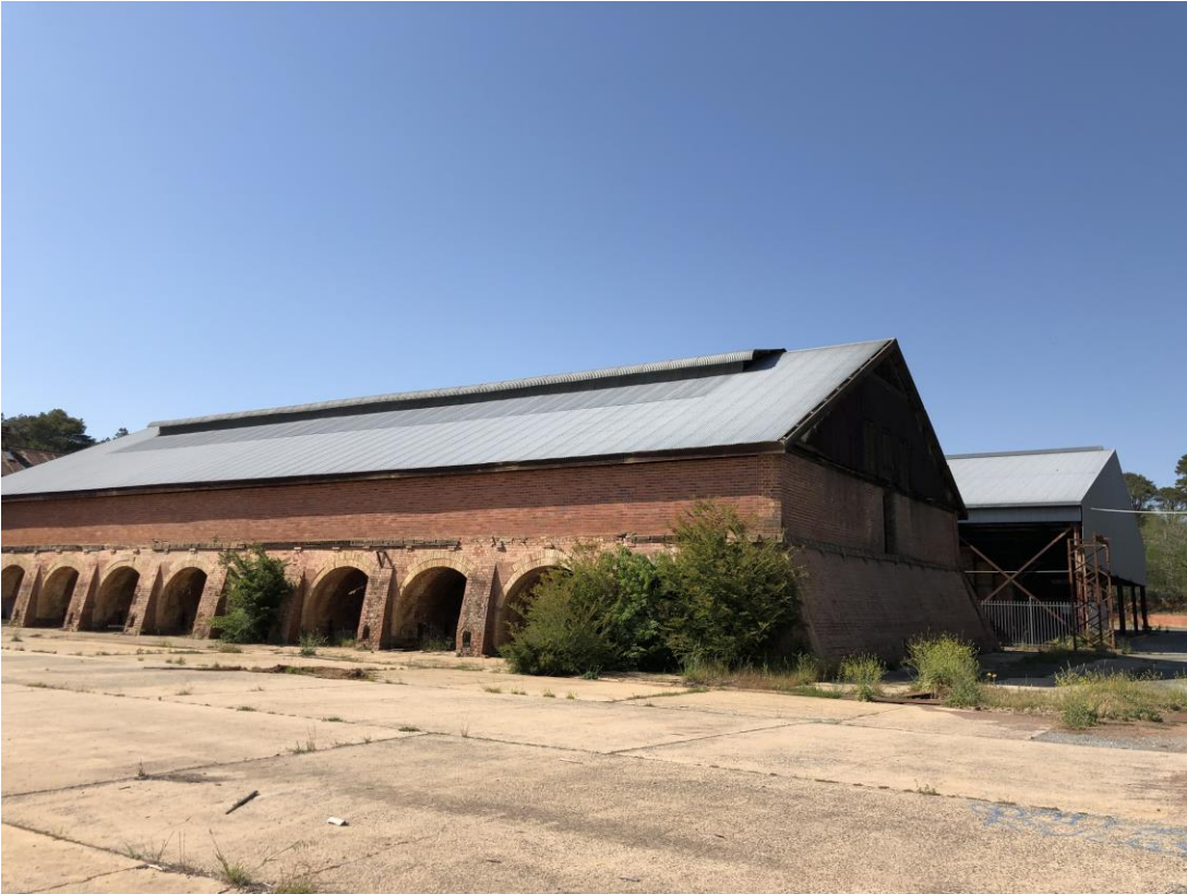
Photo 2.2 Staffordshire Kiln from Original Brickyard with overgrown vegetation (Umwelt, 2020)
