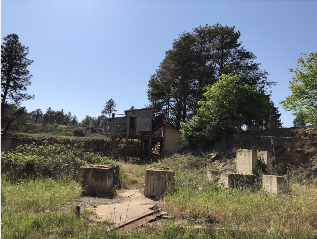
Photo 2.4 Primary Crusher Room with overgrown vegetation and scattered remnants (Umwelt, 2020)
