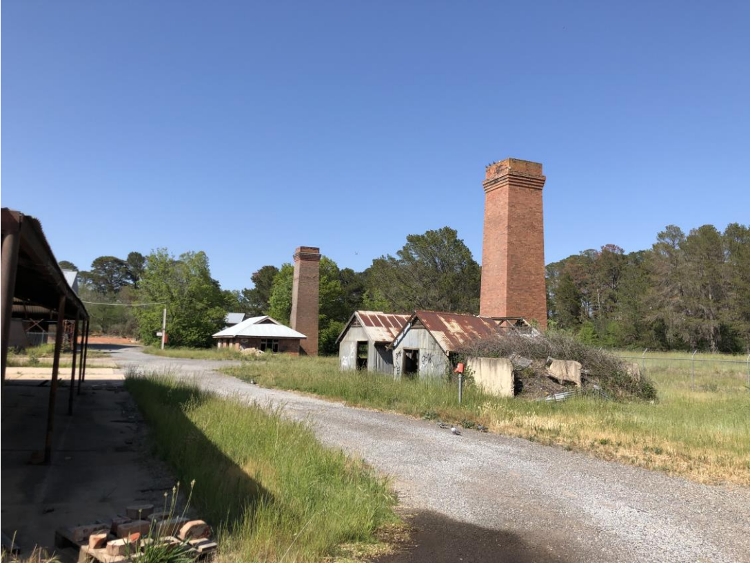
Photo 2.3 Fan House for Hardy Patent Kiln 1 in dilapidated state (Umwelt, 2020)
