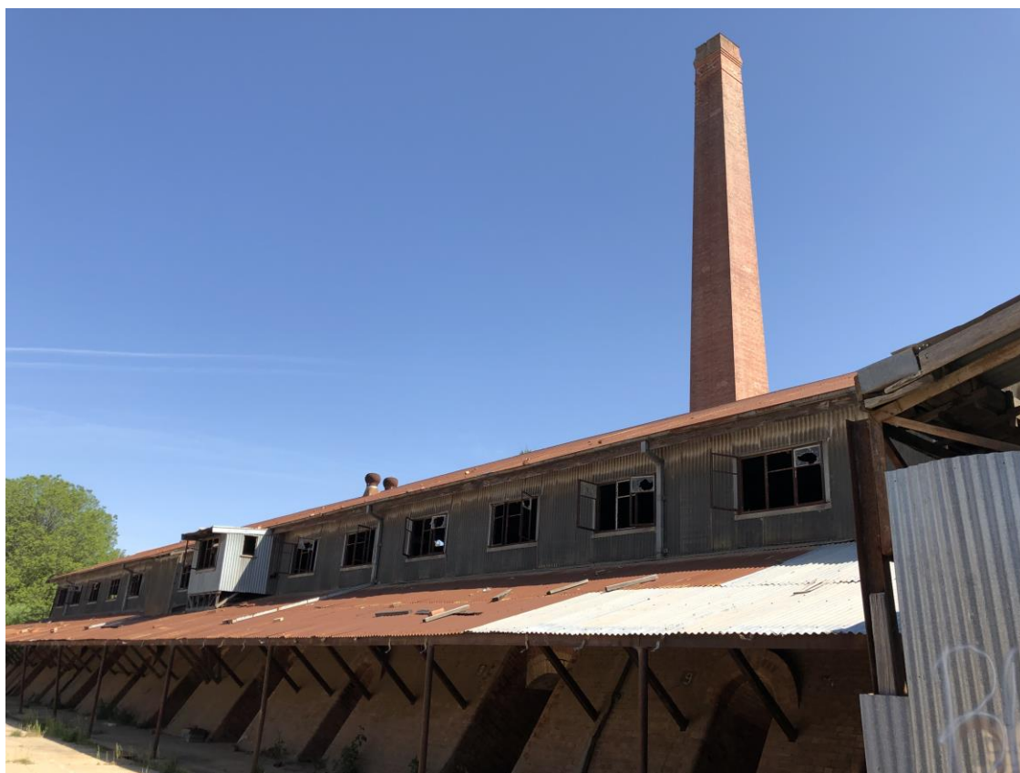
Photo 2.1 Hardy Patent Kiln 2 with signs of vandalism (Umwelt, 2020)
