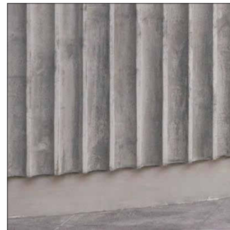
CF3 CONCRETE RIBBED
