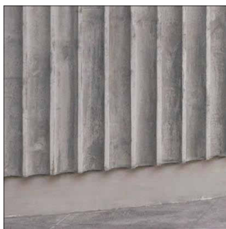
CF3 CONCRETE RIBBED
