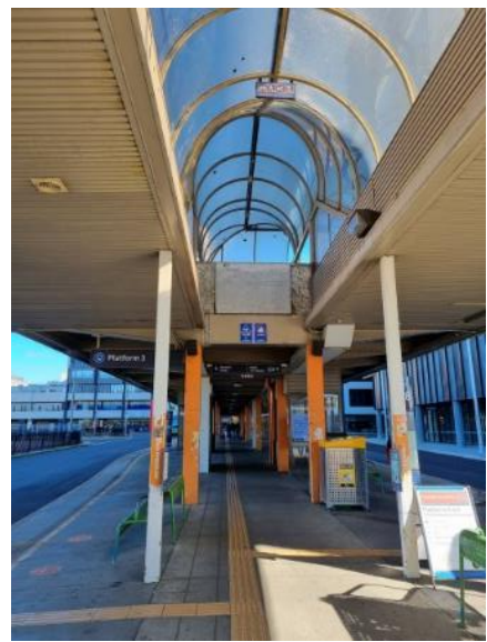
Figure 27 – Intersection of stage 1 and 2 constructions
