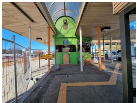
Figure 25 – View toward former ticket office
