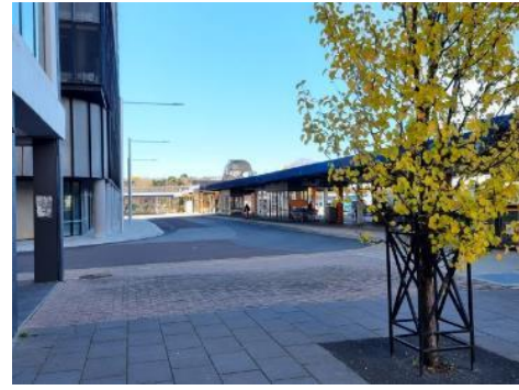
Figure 23 – East Side of east-west arm. Note overshadowing of site.
