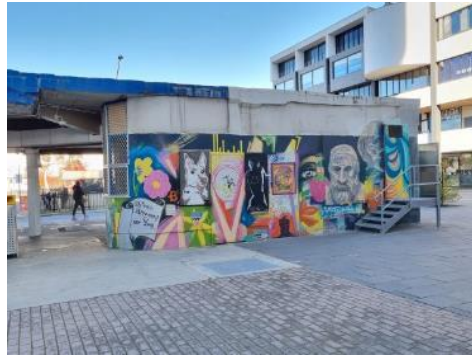
Figure 22 – Former Ticket Office building
