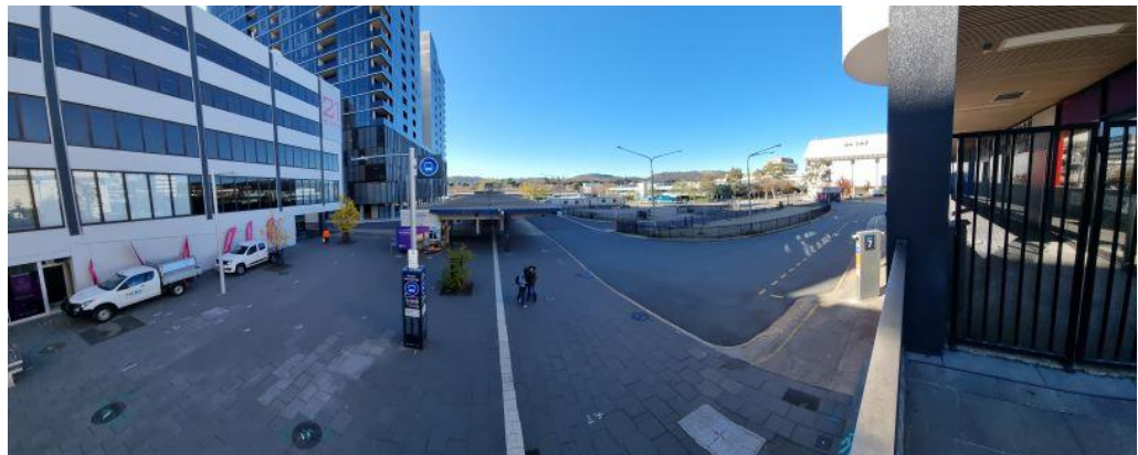
Figure 35 : Panorama of the Interchange from Woden Town Square indicating extent of overshadowing issue – June 2022
