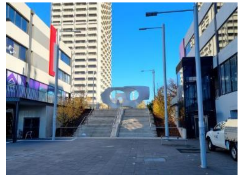
Figure 21 – New stairs to town square
