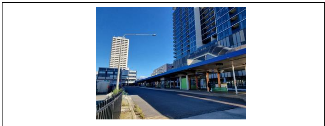
Figure 17 : East west arm of interchange showing two stages of construction in canopy
