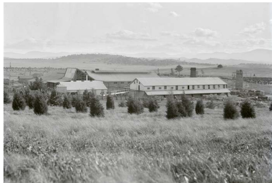
View from the north-east towards the brick processing buildings, c. 1927
