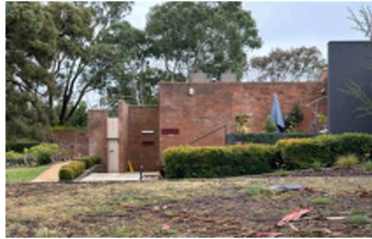
Original face brick walls to the crematorium which also contains the toilets
