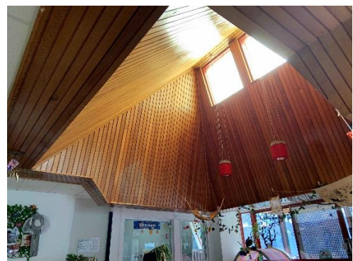
Figure 9 – Original Skylight and lining retained
