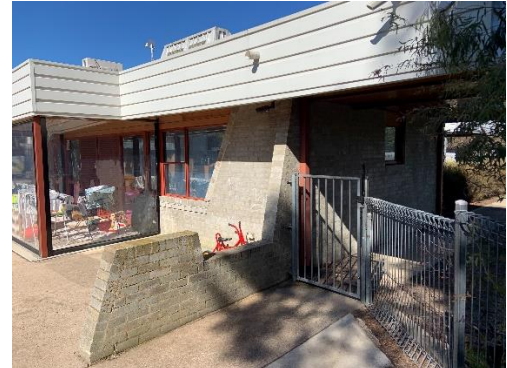
Figure 7 – Detail view of corner to be Impacted
