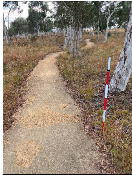
Plate 4. Previous impacts from constructed pathway.
