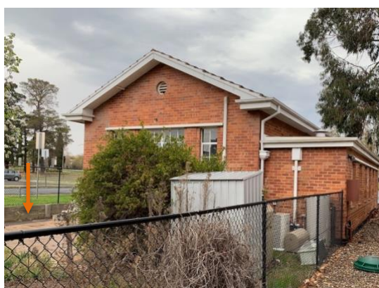
Brick paving, mesh fence, treated pine retaining wall (arrow) and metal shed to north-east of the 1948 Switch Room
