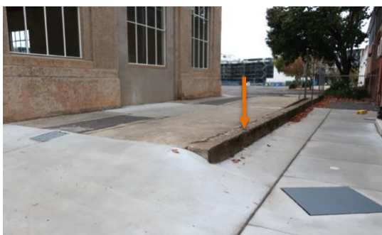
Platform wall between Fitters' Workshop and Former Transport Depot surrounded by a variety of modern pavement types
