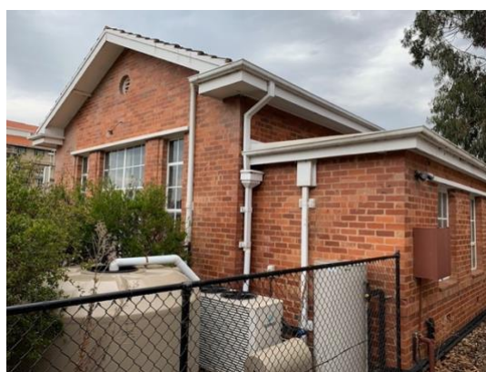
Rainwater tank to the north-east of the 1948 Switch Room
