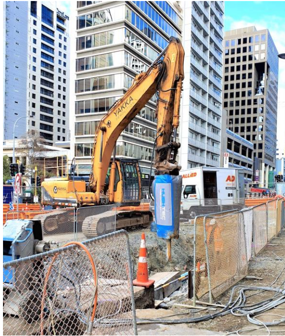
Figure 3.11 Example of noise reduction treatment on a rock-breaking head fitted to an excavator
