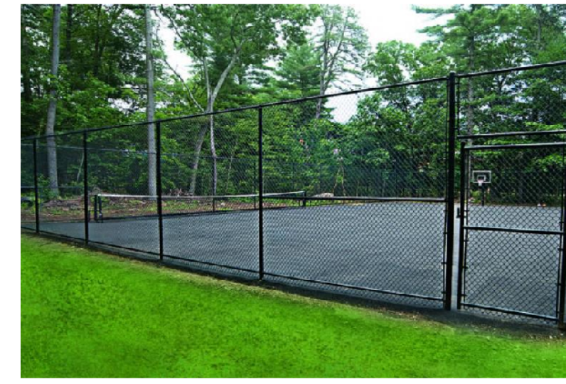
Tennis Court Fence & Entry
