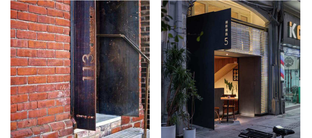
SIGNAGE TYPE 4 - DOOR REVEAL Protruding metal signboard, fixed to mullion Non illuminated
