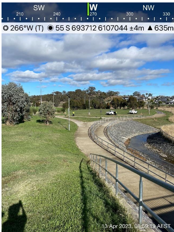
Figure 5: General view of the southern portion of the site, from the eastern end of the Bicentennial National Trail with a rock pitching drain.
