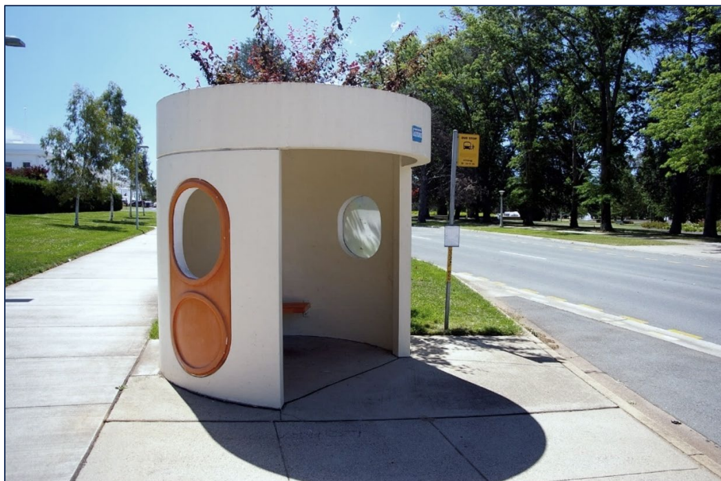
Figure 14: Canberra traditional bus shelter form
