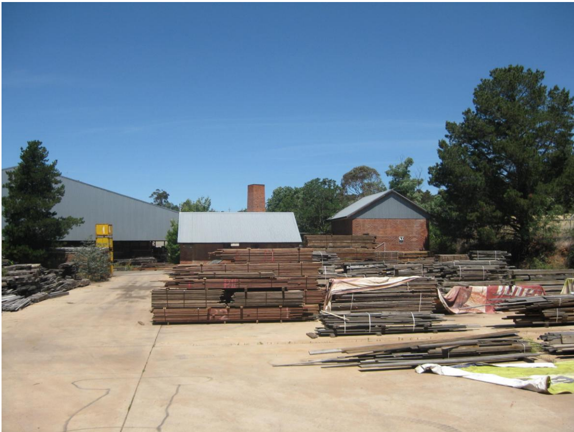
Figure 43 View looking east over the extrusion plant, part of the northern extension to the railway reserve Source: Lovell Chen
