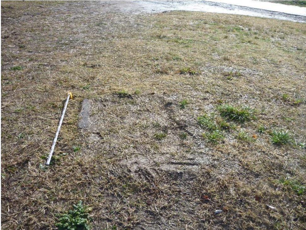
Figure 17 View of BRW1 concrete feature, looking north Source: NOHC
