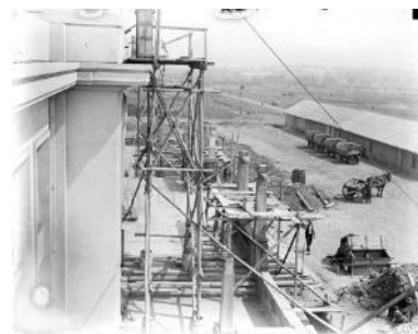
Figure 2.11 View from Old Parliament House roof with the railway and carts that delivered the bricks in the top right. (Source: NAA, A3560, 1398)
