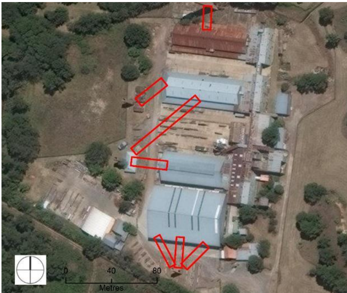
Figure 3.26 A current aerial showing the location of BRW12. (Source: ESRI Basemaps and GML Overlay)
