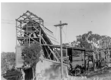
Figure 2.16 Stone crushing and screening plant. (Source: NAA, A3560)
