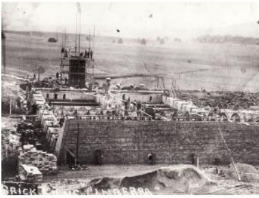
Figure 2.5 Staffordshire kiln construction at the Brickworks, c1915. (Source: Canberra District Historical Society, ID15652)
