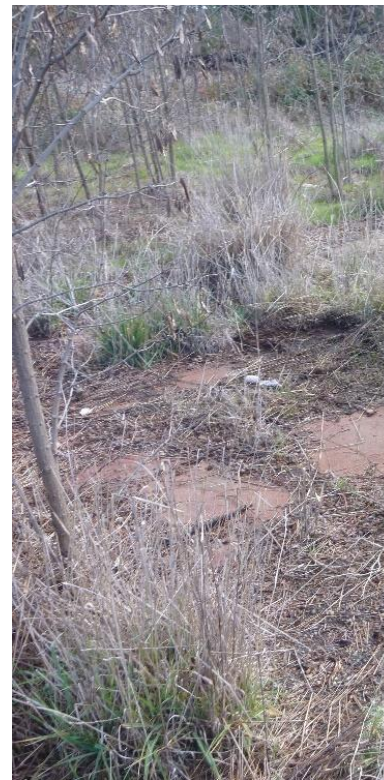
Figure 23 The concrete slab at Source: NOHC
