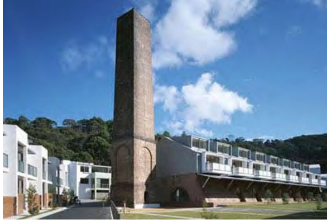
Figure 2.30 The adapted/redeveloped kiln and truncated stack at Brookvale Brickworks. (Source: < www.marchesepartners.com.au >)
