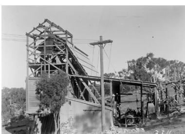
Figure 2.16 Stone crushing and screening plant. (Source: NAA, A3560)
