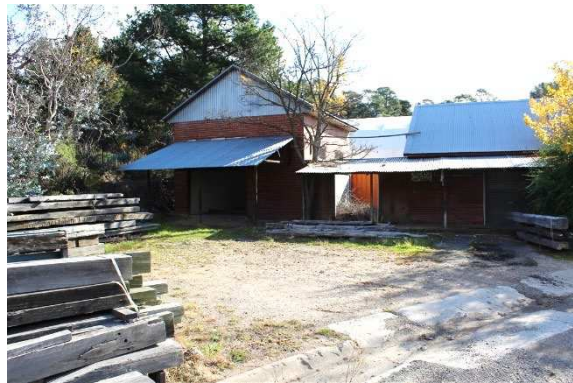
Figure 3.26 Boiler House (Element 30) and Substation/Control Room (Element 29). (Source: GML, 2017)
