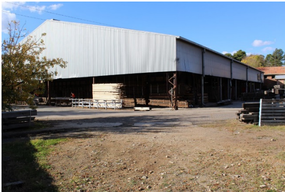
Figure 3.9 Downdraught Kilns (Element 6) beneath steel Canopy. (Source: GML, 2017)
