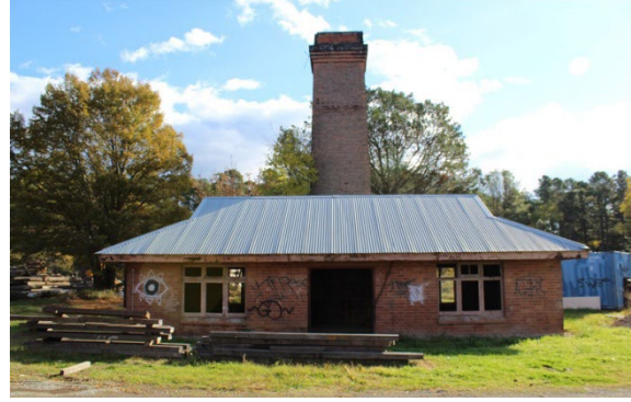
Figure 3.14 Fan House (Element 2) and Chimney Stack (Element 7) for Staffordshire Kiln. (Source: GML, 2017)
