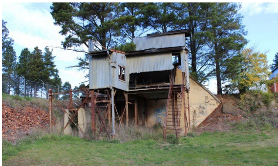
Figure 3.18 Primary Crusher House (Element 20). (Source: GML, 2017)
