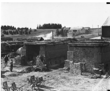
Figure 2.7 Scotch kilns were in operation at the Brickworks till the mid-1920s. (Source: NAA, A3560, 1968)
