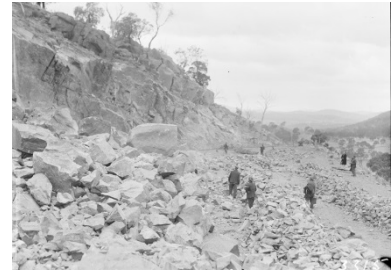
Figure 2.9 The Brickworks quarry face with workers, c1920–30. (Source: NAA, A3650, 3315)
