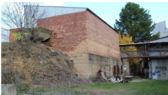
Figure 3.34 Concrete retaining wall (Element 24), showing later masonry wall constructed on top. (Source: GML, 2017)
