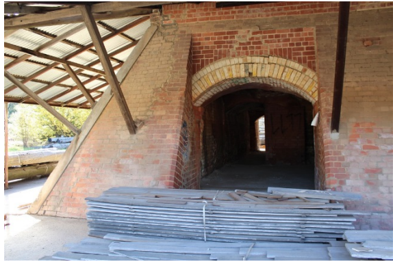
Figure 3.6 Brickwork and verandah detailing of Hardy patent kiln 1 (Element 3). (Source: GML, 2017)
