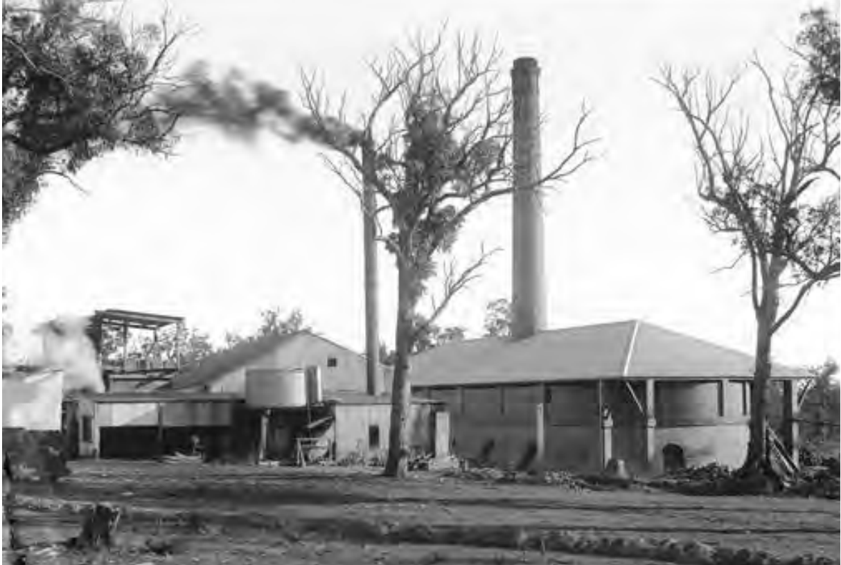
Figure 2.46 Armadale Brickworks c1905. (Source: State Library of WA)
