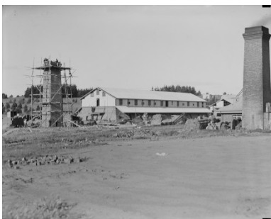
Figure 2.6 Chimney stack under construction, c1926. (Source: NAA, A3560, 2455)
