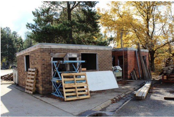
Figure 3.25 Ancillary Storage Building (Element 28) and Amenities Building 2 (Element 31). (Source: GML, 2017)
