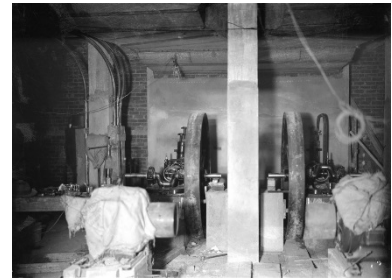
Figure 2.18 Brick pressing machinery being installed at the Brickworks, c1925. (Source: NAA, A3560, 1210)
