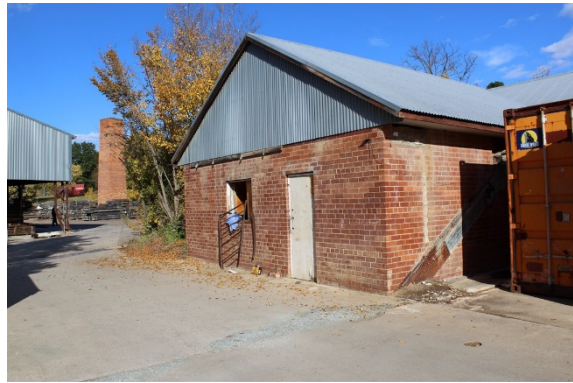
Figure 3.28 Substation/Control Room (Element 29). (Source: GML, 2017)
