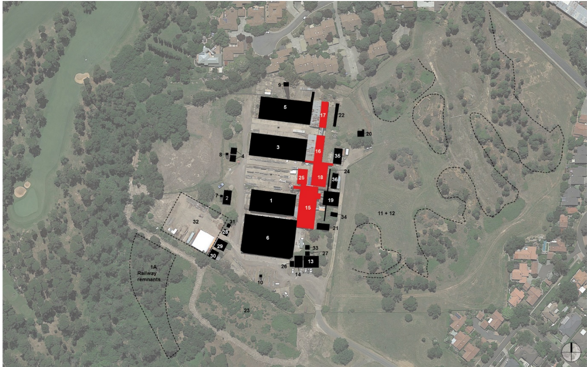
Figure 3.16 Location of the machine bays and workshop at the site, shown in red. (Source: Google Earth with GML overlay, 2017)
