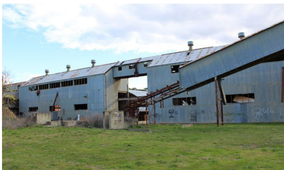
Figure 3.20 Machine Bay 2/3 (Elements 16/17) with Elevator/Conveyor (Element 22) in foreground. (Source: GML, 2017)
