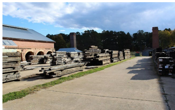
Figure 3.38 First brickyard (Element 37), looking west. (Source: GML, 2017)
