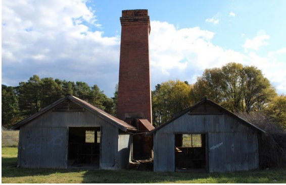
Figure 3.13 Fan Houses (Element 4) and Chimney Stack (Element 8) for Hardy Patent Kiln 1. (Source: GML, 2017)
