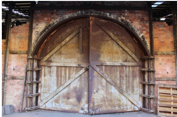
Figure 3.10 Door of a Downdraught Kiln. (Source: GML, 2017)
