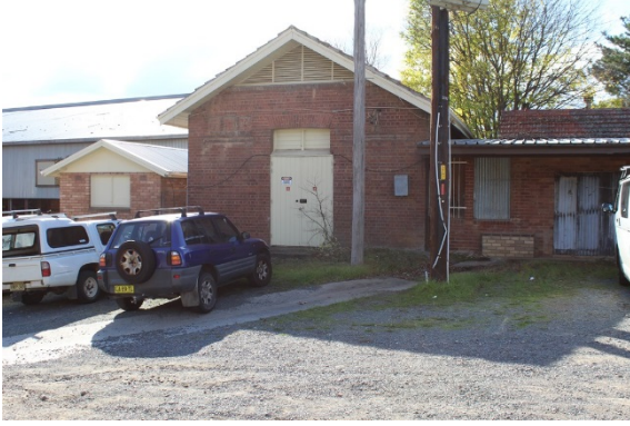
Figure 3.23 Control Room (Element 26), Power House (Element 14), and Office (Element 13). (Source: GML, 2017)
