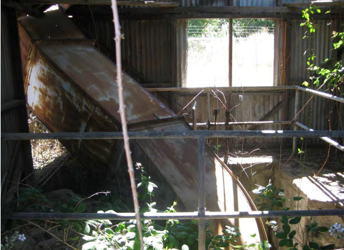
Figure 90 Interior of the 1927 fan house.
