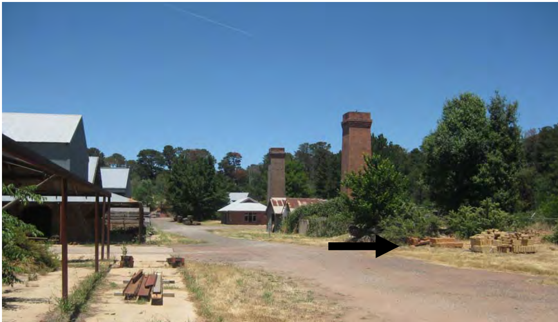
Figure 161 The approximate site of the former forklift shed indicated by the arrow.
