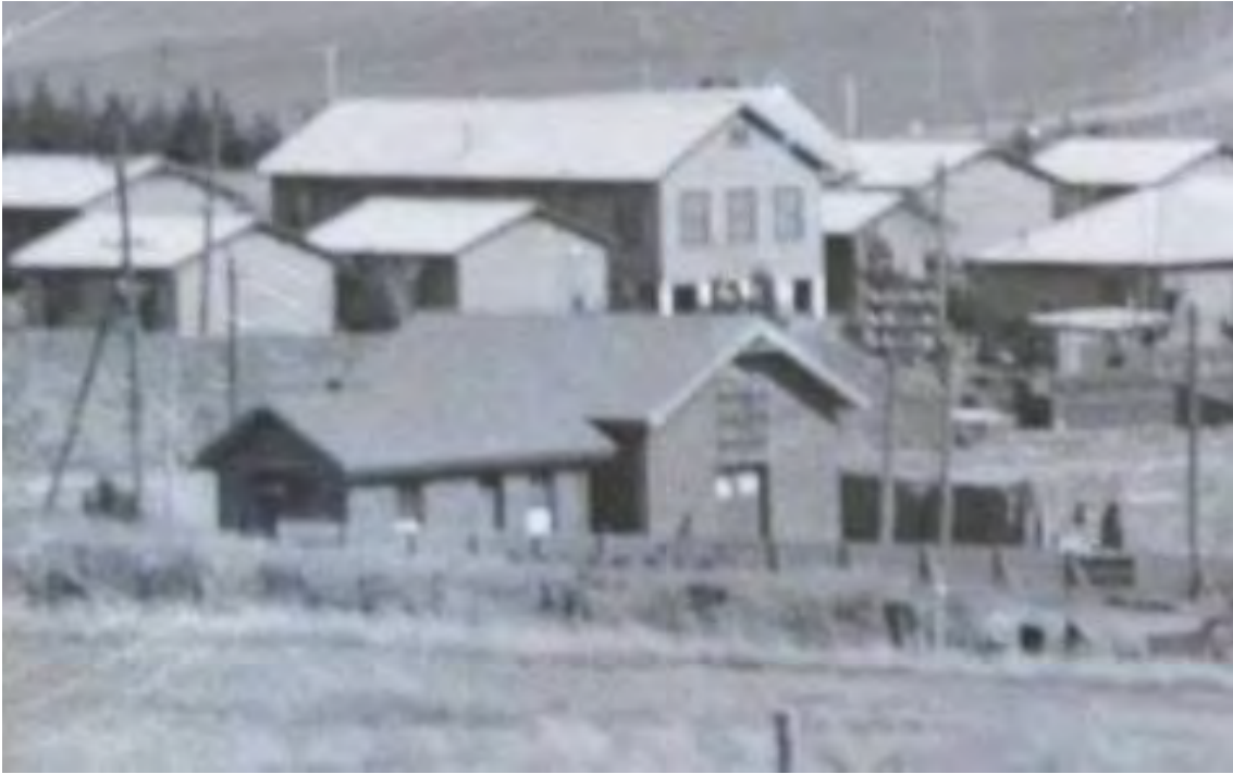
Figure 79 Detail of a photograph of the Brickworks site in 1929 taken from the quarry area, showing the original form of the office building to the east of the Power House (foreground). Note that at this date, the main entrance to the Power House is from the north. The married quarters camp is in the background. Source: National Archives of Australia.
