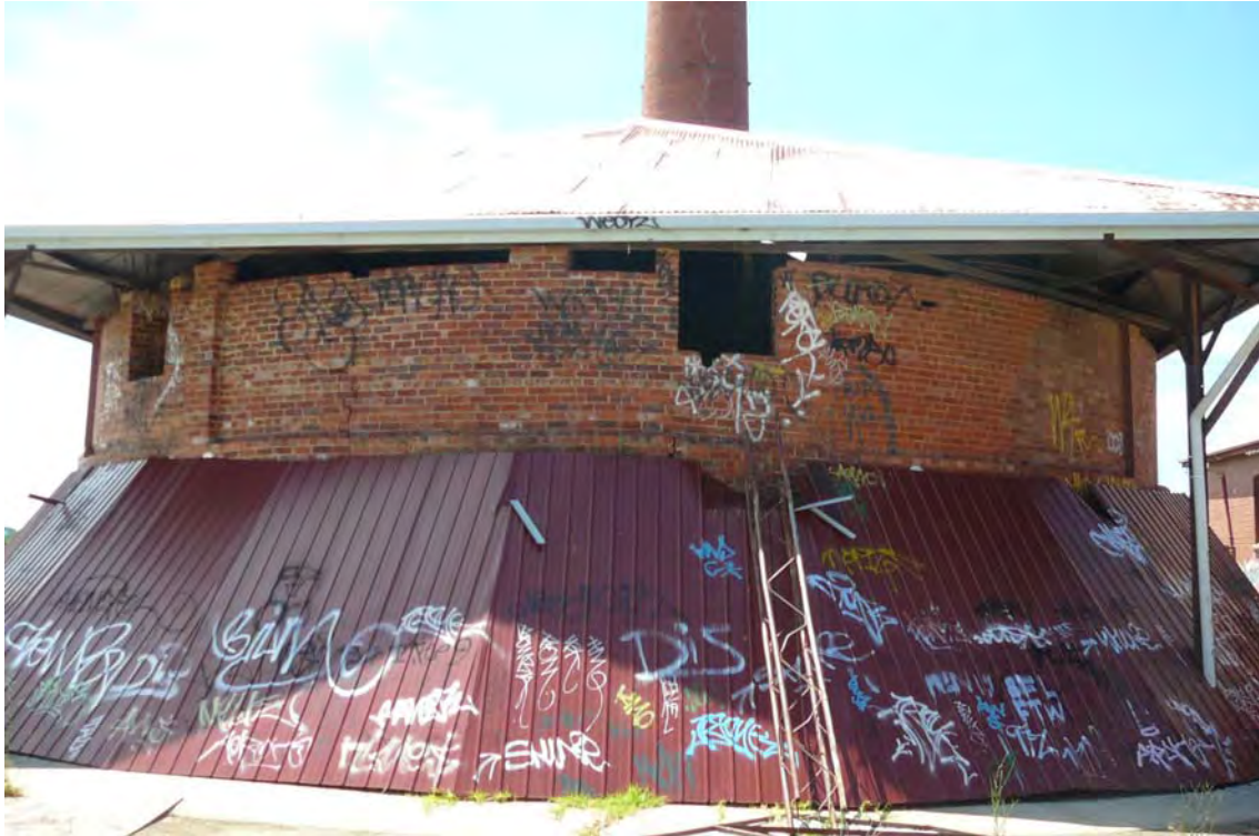
Figure 17 Hoffman kiln at the former Standard Brickworks, Box Hill (Victoria) Source: Lovell Chen, January 2010
