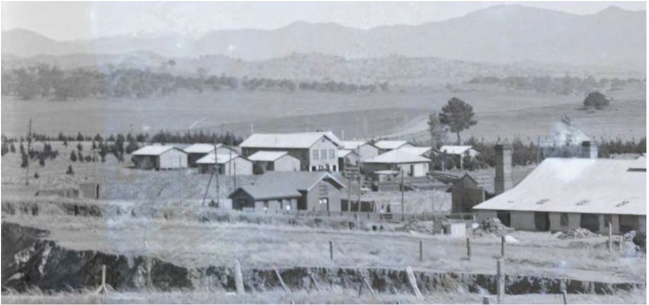
Figure 66 The married quarters camp (background), built to the south-west of the Brickworks in 1927.
