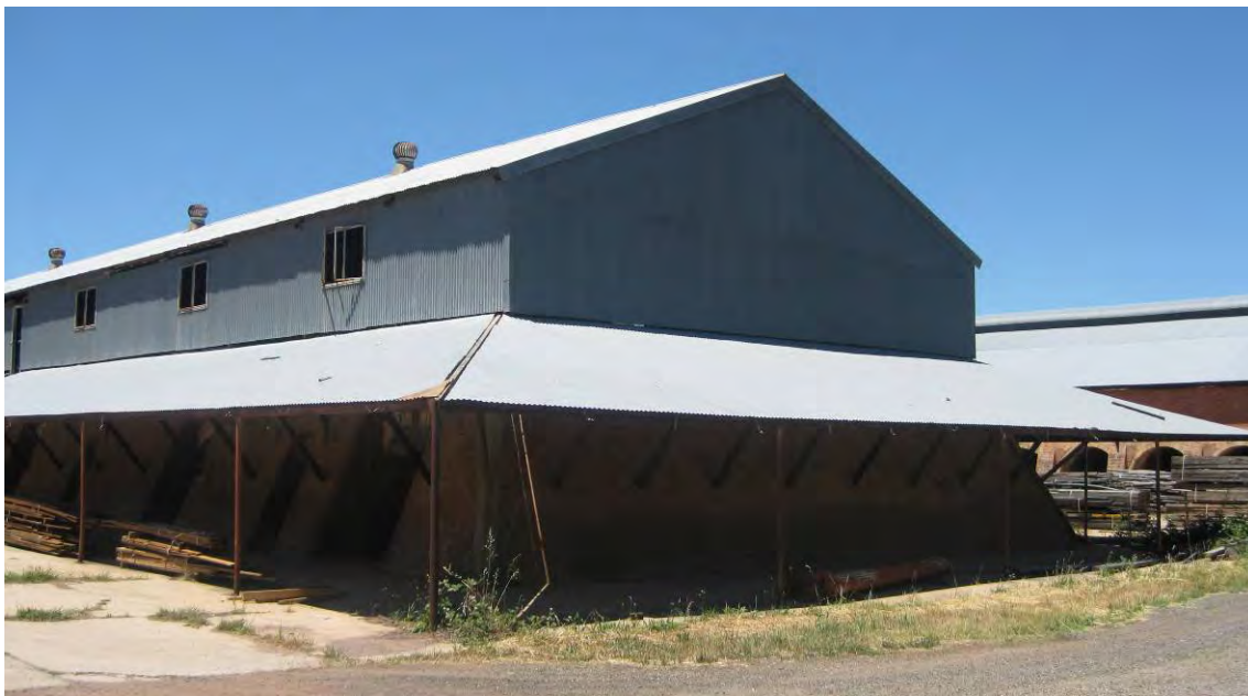
Figure 84 The Hardy patent kiln showing the west and part of the north elevation.
