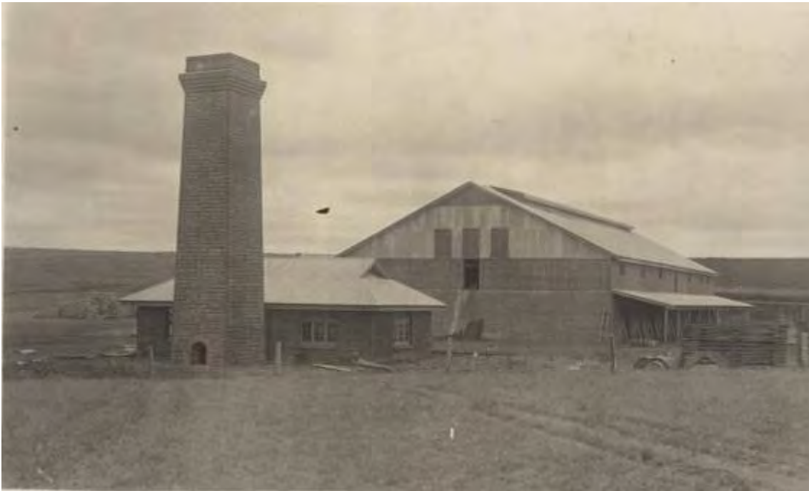
Figure 49 The Staffordshire kiln, fan house and stack, photographed in 1917 by Harry Connell. Note that in this view the kiln verandah does not extend to the west elevation.
