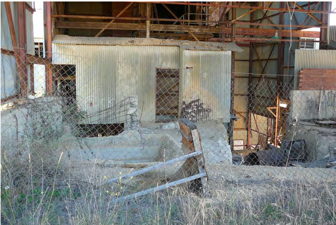
Figure 127 Interior of the White Pan Room looking west. The site of the now-removed hoppers is in the foreground.
