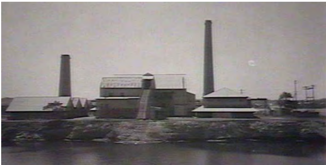
Figure 170 Continuous kilns at State Brickworks, pictured 1957. Source: NSW Heritage Register.
