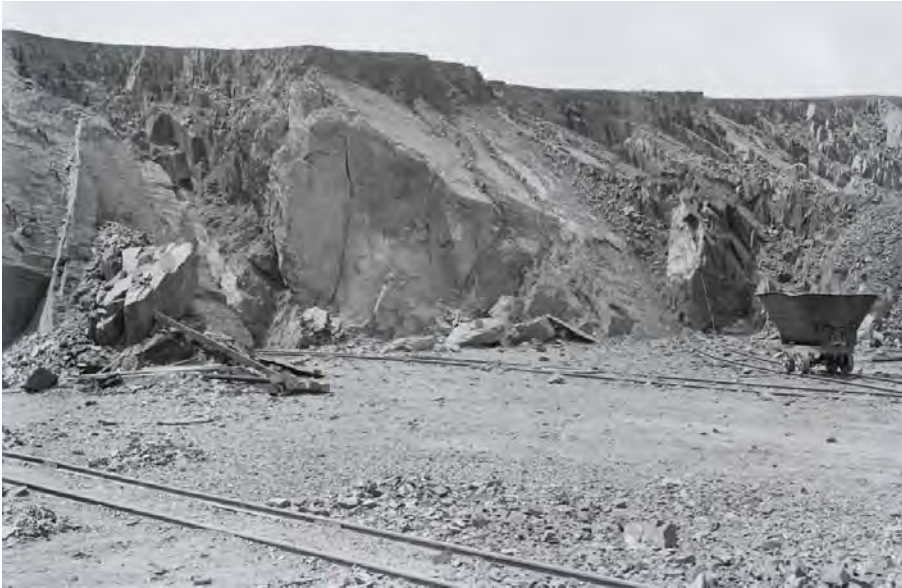
Figure 37 View of the quarry showing the narrow gauge tramway used to transport shale to the crusher, 1921. Source: National Archives of Australia.
