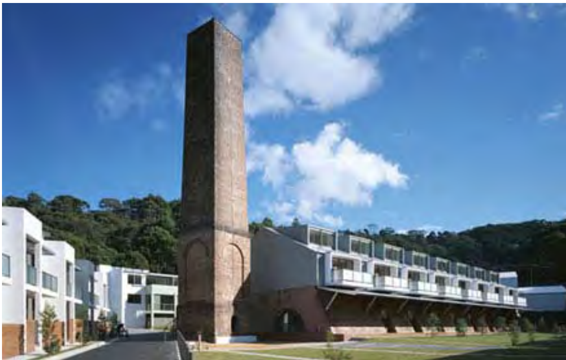
Figure 168 The adapted/redeveloped kiln and truncated stack at Brookvale Brickworks. Source: www.marchesepartners.com.au
