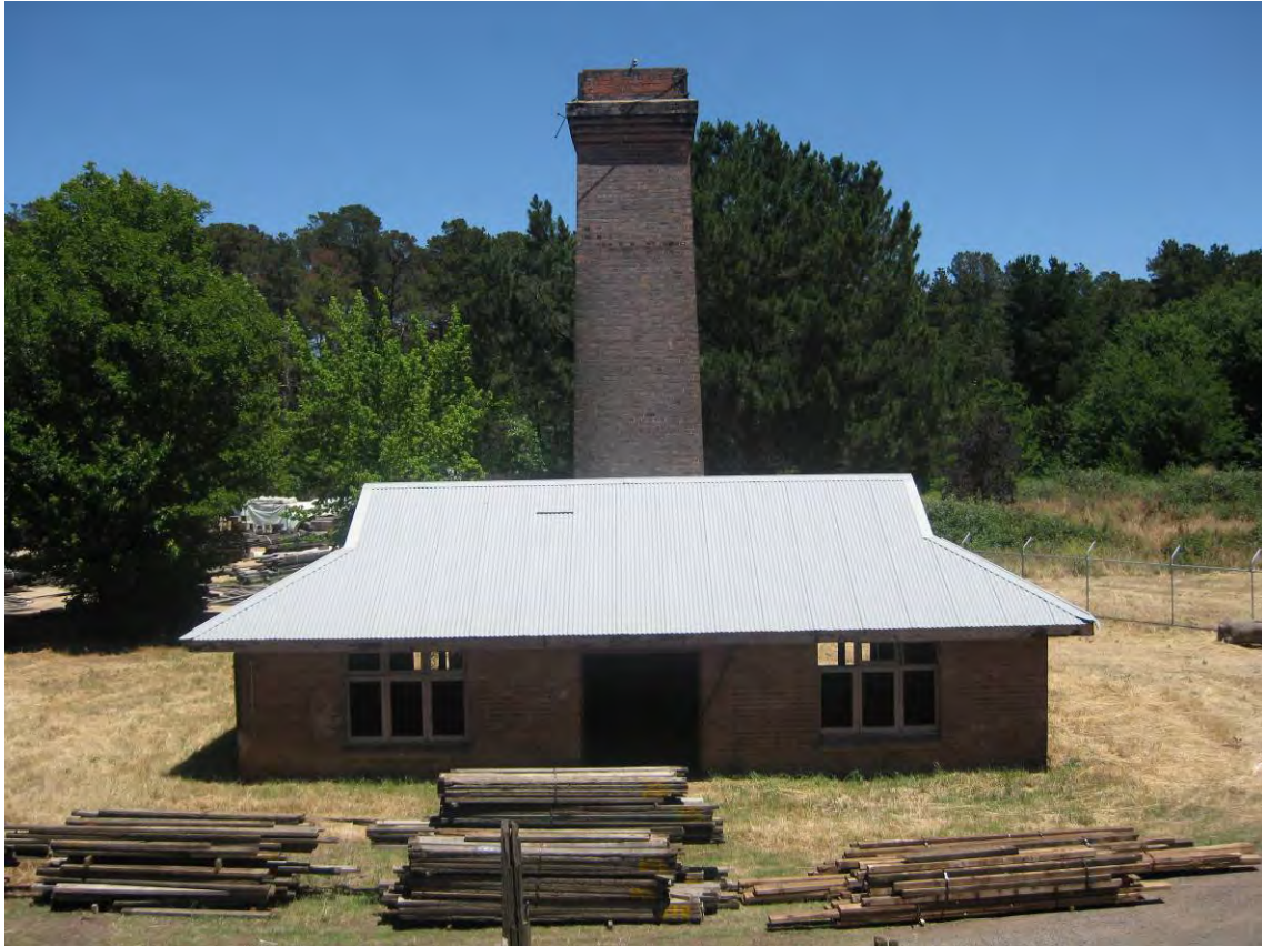
Figure 57 Fan house with stack behind.
