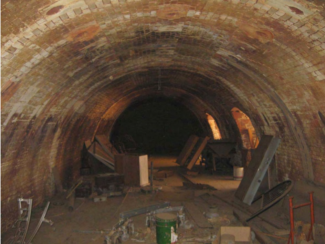
Figure 85 Interior of the Hardy patent kiln. The kiln is divided in two by a non-original brick wall.
