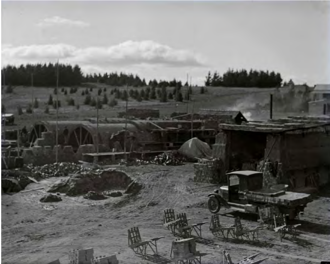
Figure 199 Hardy patent kiln under construction, looking north-east. Note the plantings on the ridge.
