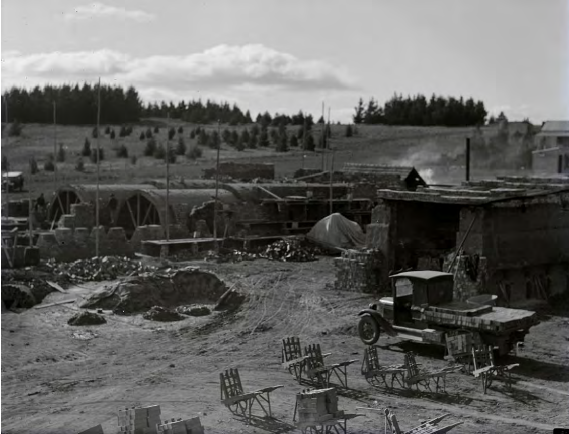
Figure 75 Hardy patent kiln under construction, 1926. Note Scotch kiln to right of picture. Source: National Archives of Australia.
