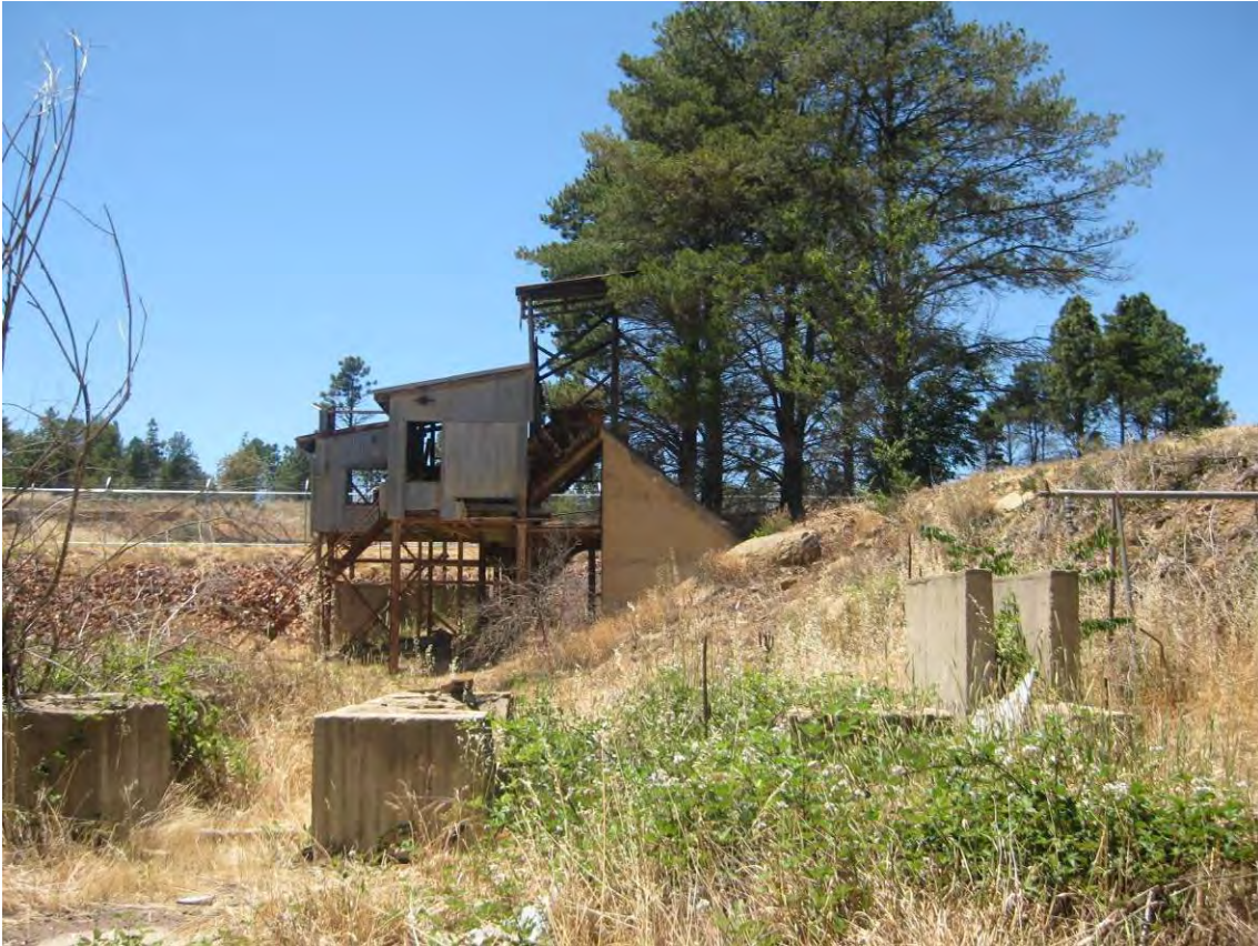
Figure 130 The Primary Crusher House viewed from the west. The concrete footings in the foreground supported the now demolished conveyor which transported crushed material to the Red Pan Room (also demolished) for further refining.
