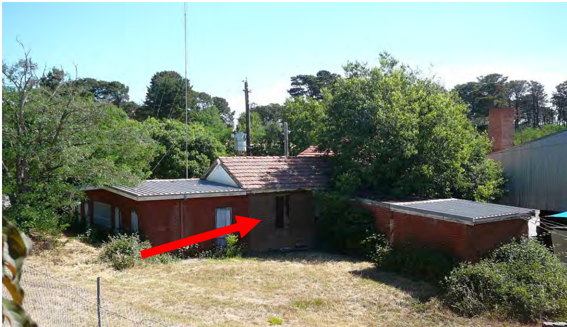
Figure 81 East and north elevations, showing the extent of the additions. The only portion of the original two-roomed structure, not enclosed by additions is indicated by the arrow.
