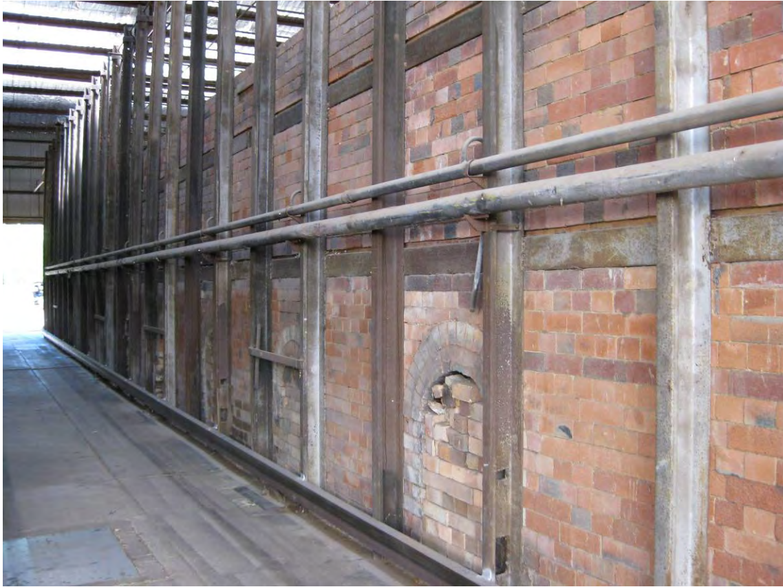
Figure 138 Side elevation showing steel framing and fireholes.
