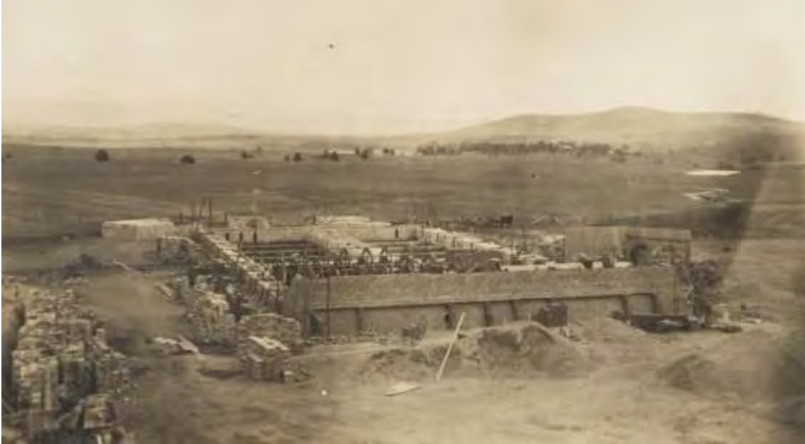
Figure 31 Staffordshire kiln under construction, c. 1915 Source: National Library of Australia.
