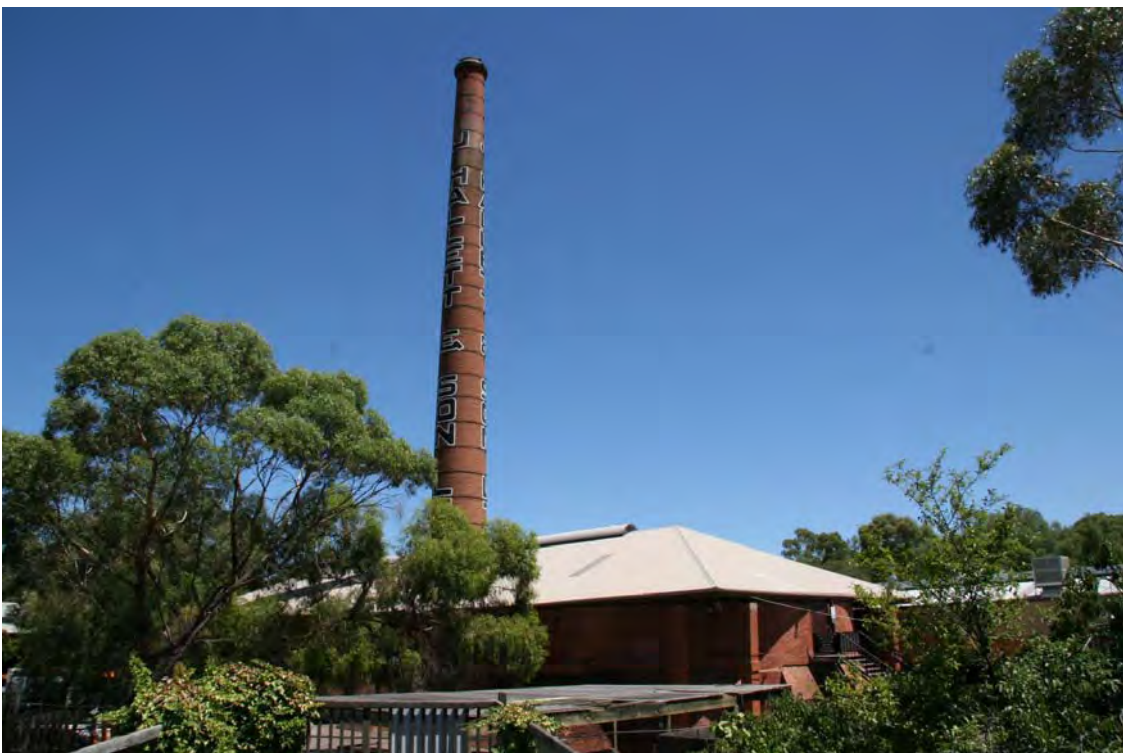
Figure 177 Brickworks Market (January 2010). Source: Lovell Chen
