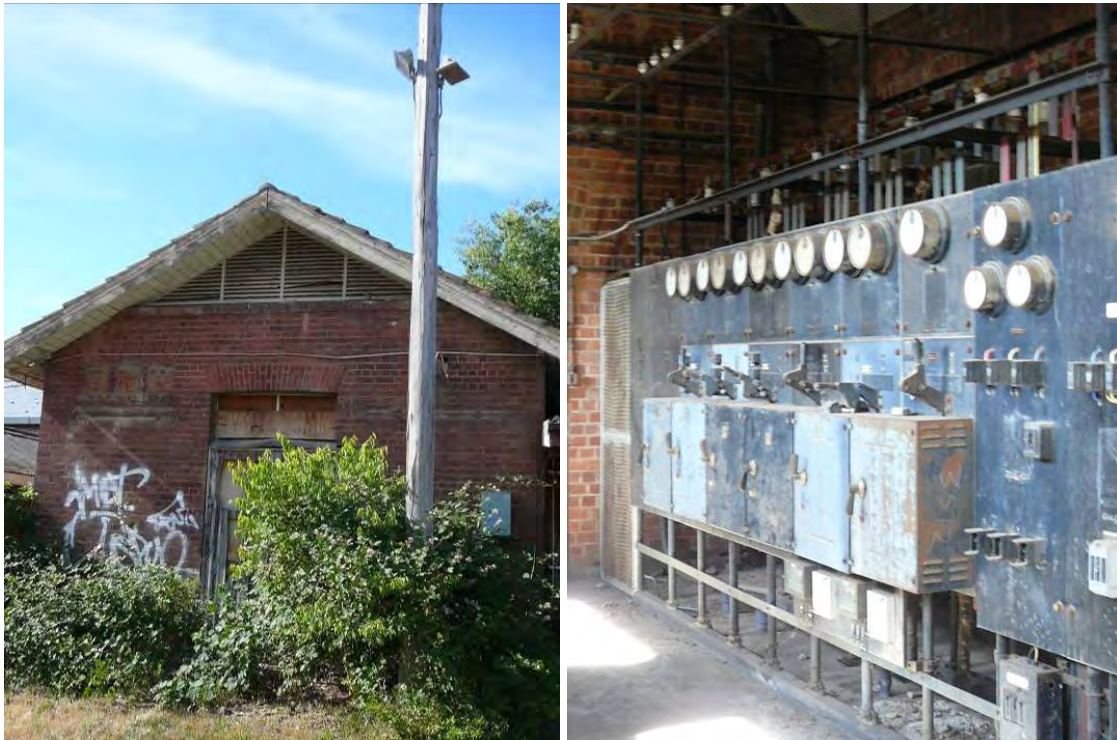
Figure 48 From left: South elevation and entry; interior showing retained plant.
