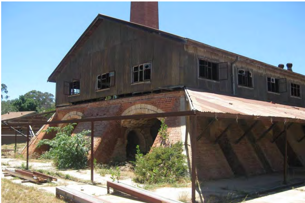
Figure 103 The Hardy patent kiln, showing the west end and part of the south elevation. Note the verandah cladding has been removed and the kiln wall part removed, presumably for improved access to the kiln interior.
