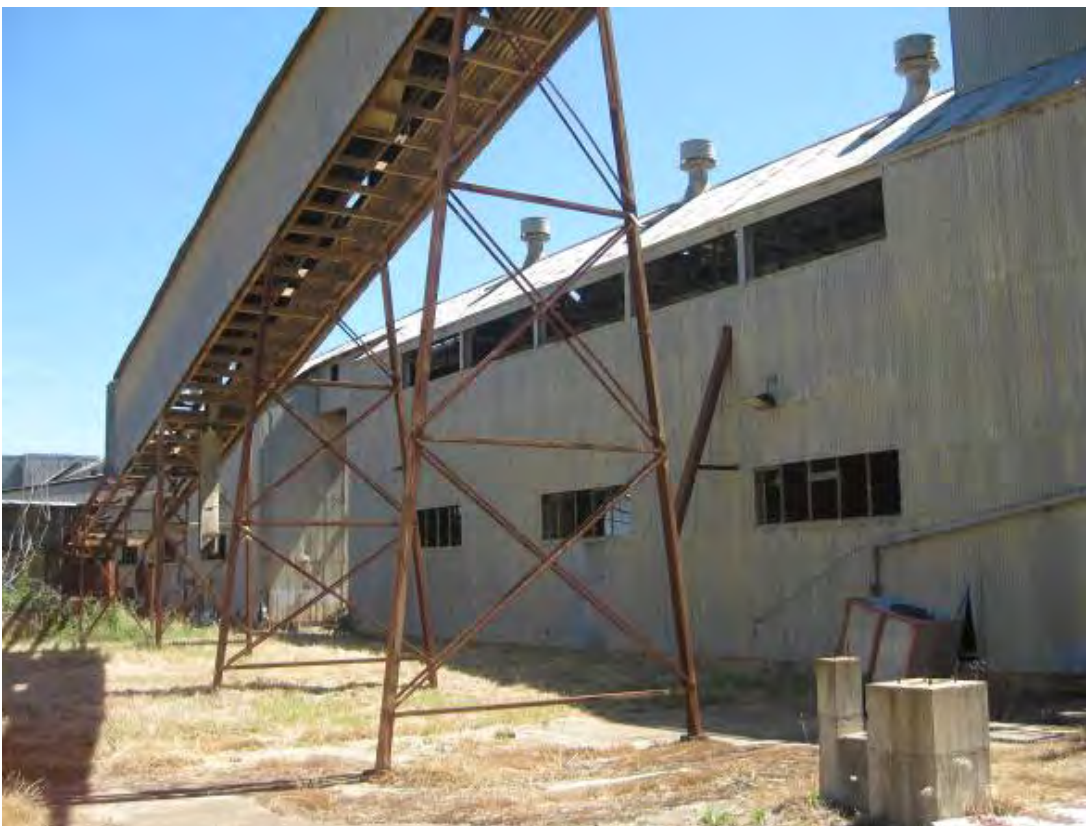
Figure 133 Looking south-west. Machine Bay III (Building 16) is in the background.
