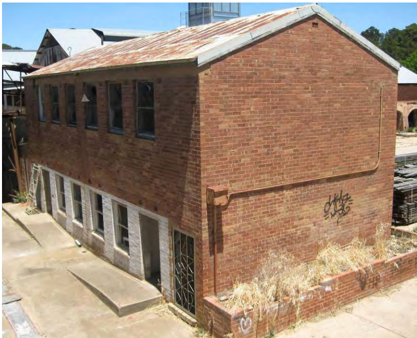
Figure 101 The Amenities Block viewed from the west.
