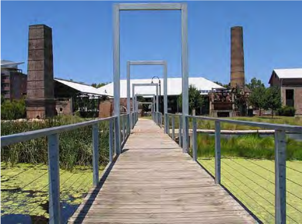
Figure 162 The Holroyd Gardens redevelopment at the former Goodlet and Smith Brickworks, pictured 2008. Source: Flickr
