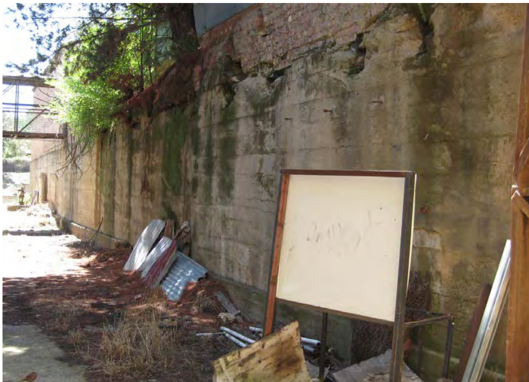
Figure 45 Retaining wall to the rear of the Workshop (Building 17).
