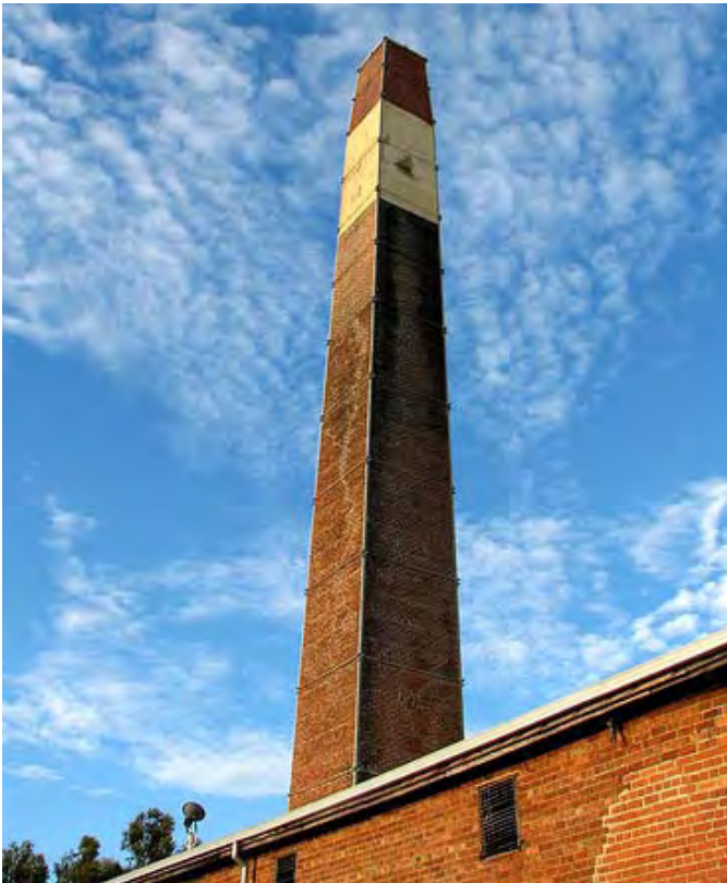
Figure 185 Recent shot of the Hoffman kiln and integrated stack at the former Maylands works. Source: Flickr
