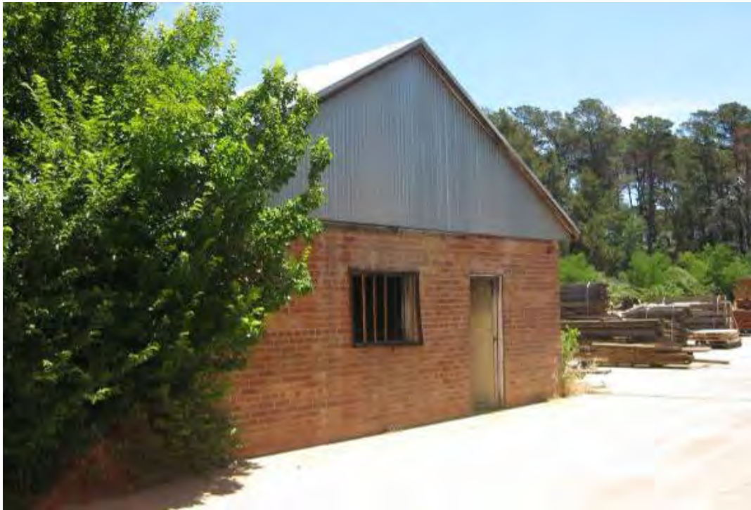
Figure 144 Substation/control room building, showing north elevation.
