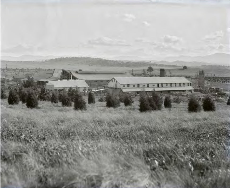
Figure 5 View from the north-east towards the brick processing buildings, c. 1927 Source: National Library of Australia.
