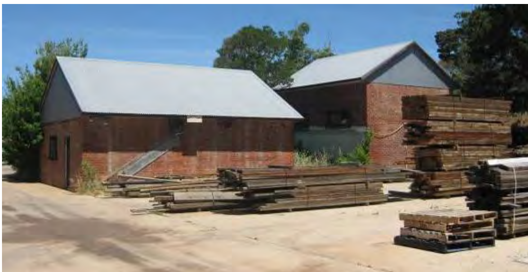
Figure 145 The former boiler house and adjoining substation/control room, photographed from the site of the former extrusion plant. The substation building is at left.
