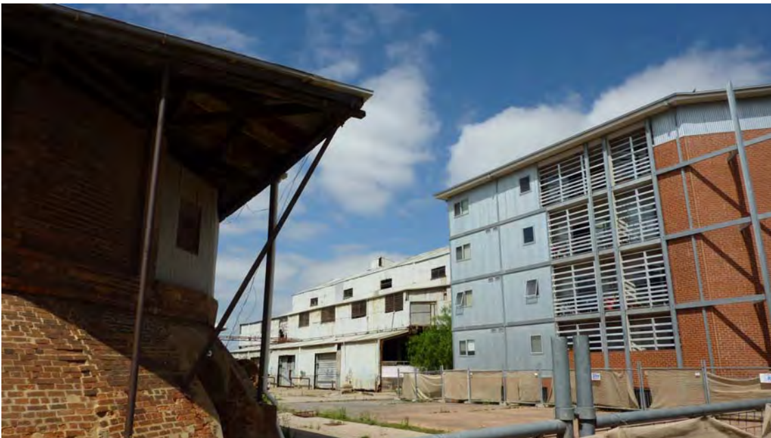
Figure 180 Former Hoffman works at Brunswick, pictured January 2010. Source: Lovell Chen.
