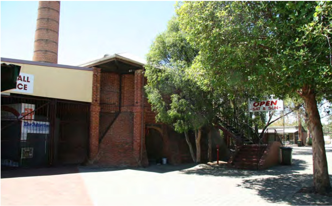
Figure 176 Brickworks Market (January 2010). Source: Lovell Chen
