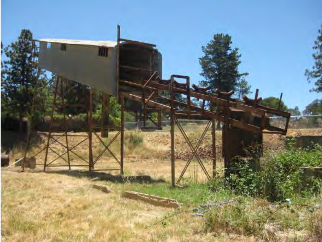
Figure 132 Extant section of the elevator/conveyor looking north-east.
