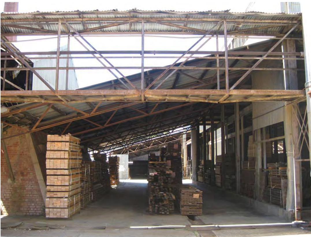
Figure 111 Interior of the Machine Bay II shop floor, looking north.
