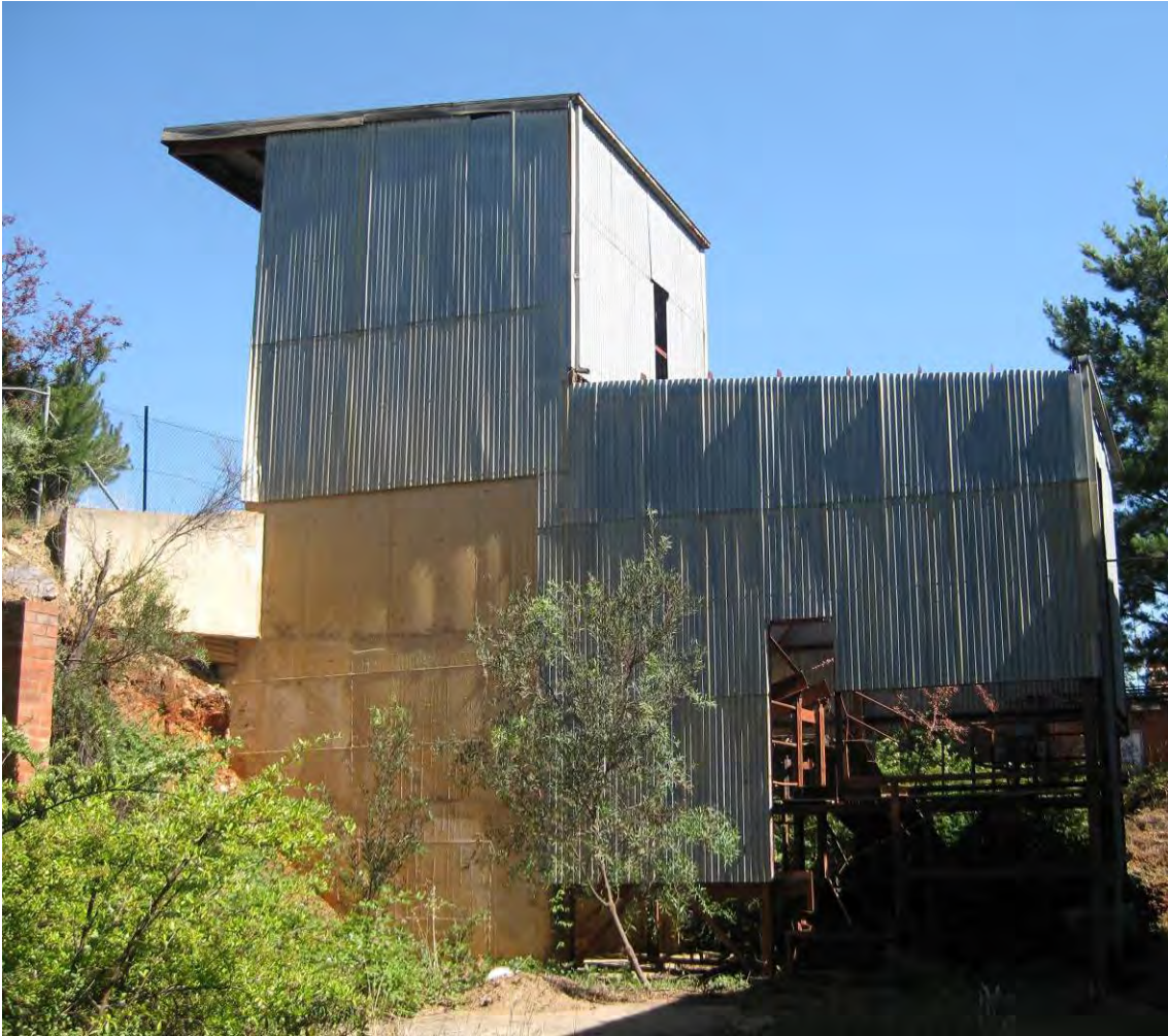
Figure 124 Small Crusher House viewed from the north.
