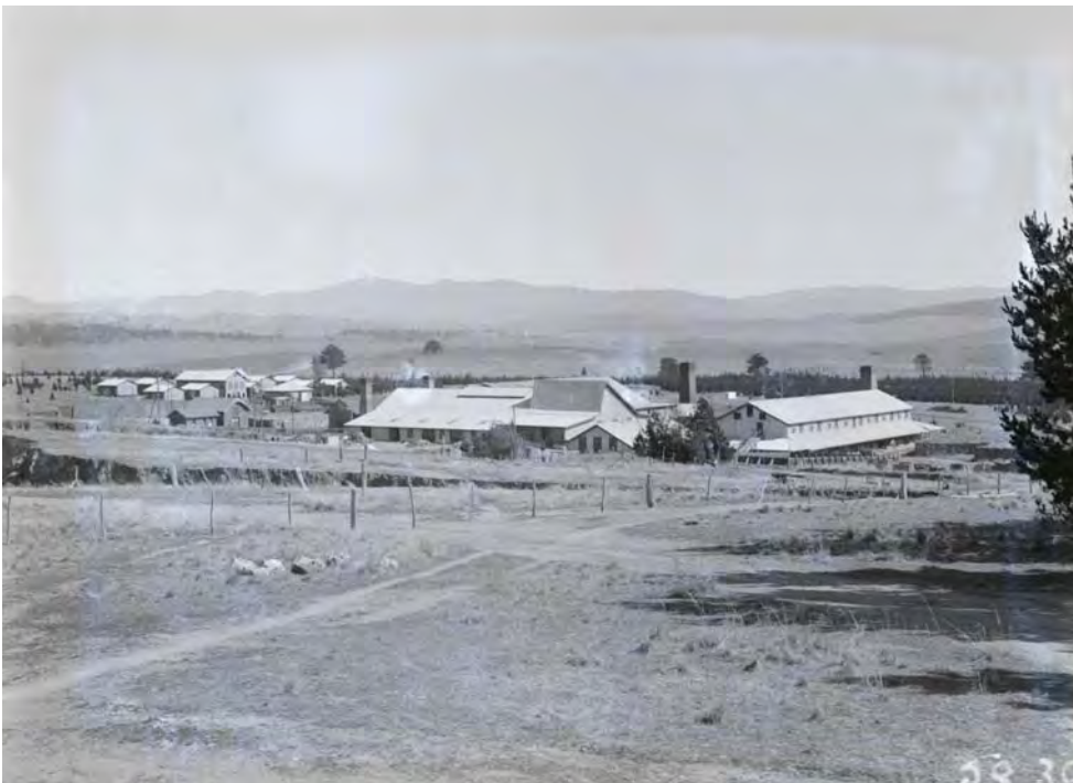
Figure 6 Another view, c. 1927. Note the excavated quarry on the left. Source: National Library of Australia.
