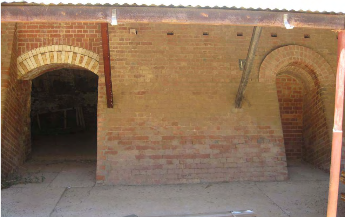
Figure 86 Kiln wickets – the opening at left has been altered to enable forklift access and the bricked-up the opening at right is as originally built.
