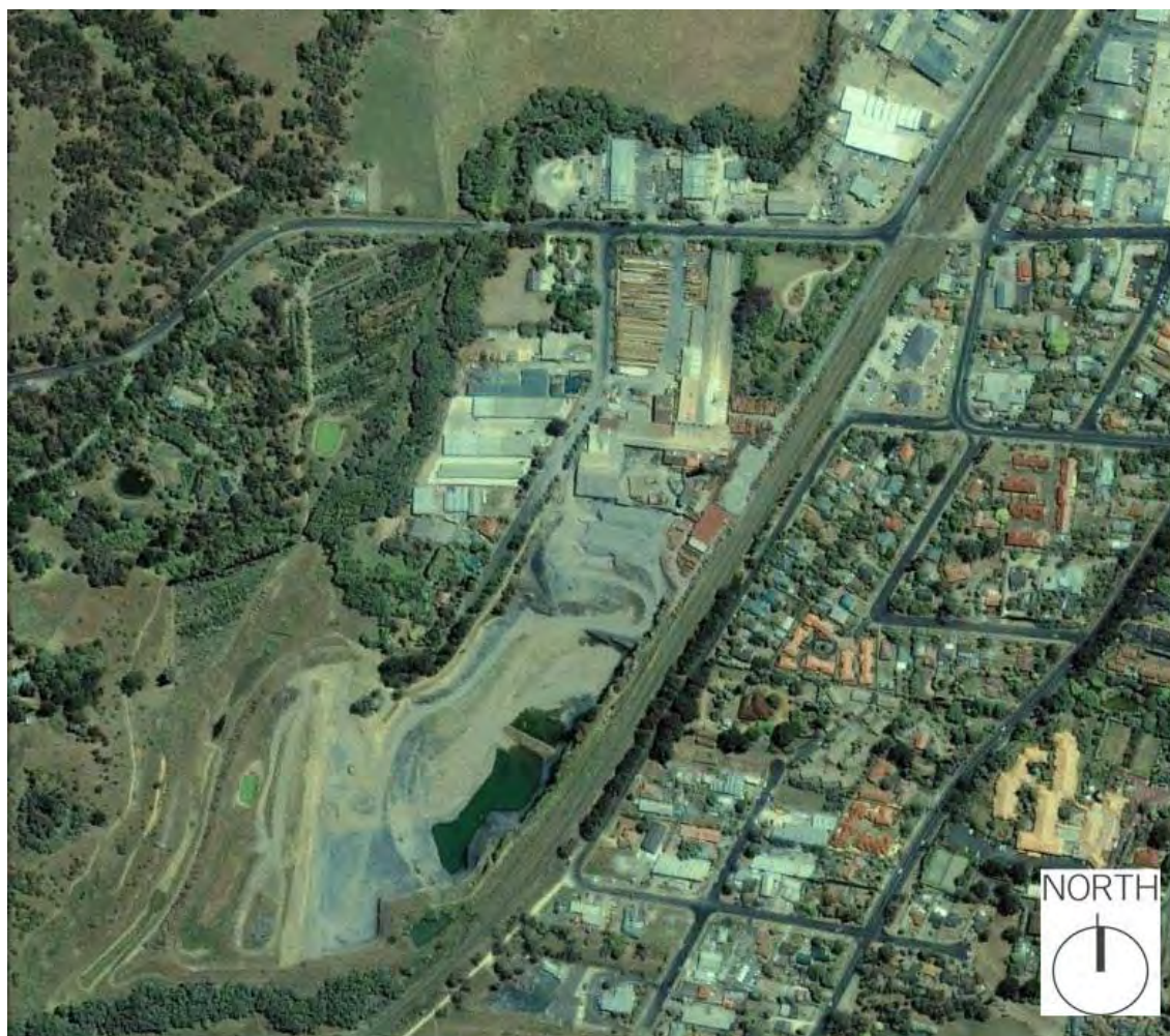
Figure 172 Recent aerial view of Bowral Bricks.
