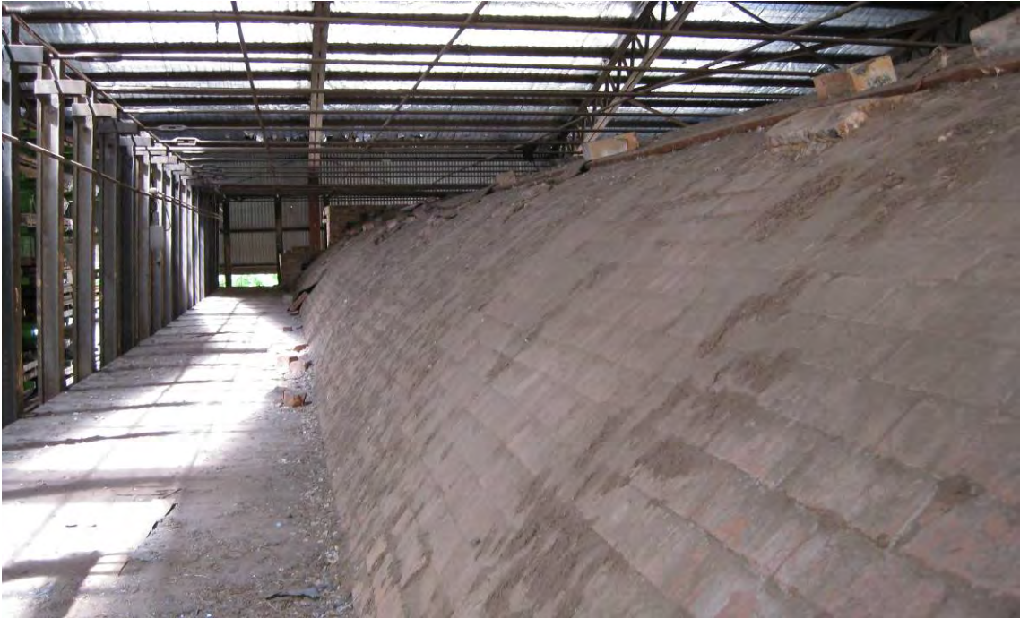
Figure 136 Kiln roof with brick walkway to sides.
