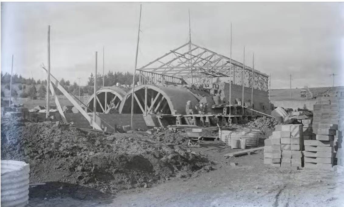
Figure 76 Hardy patent kiln under construction, c. 1926. Source: National Archives of Australia.
