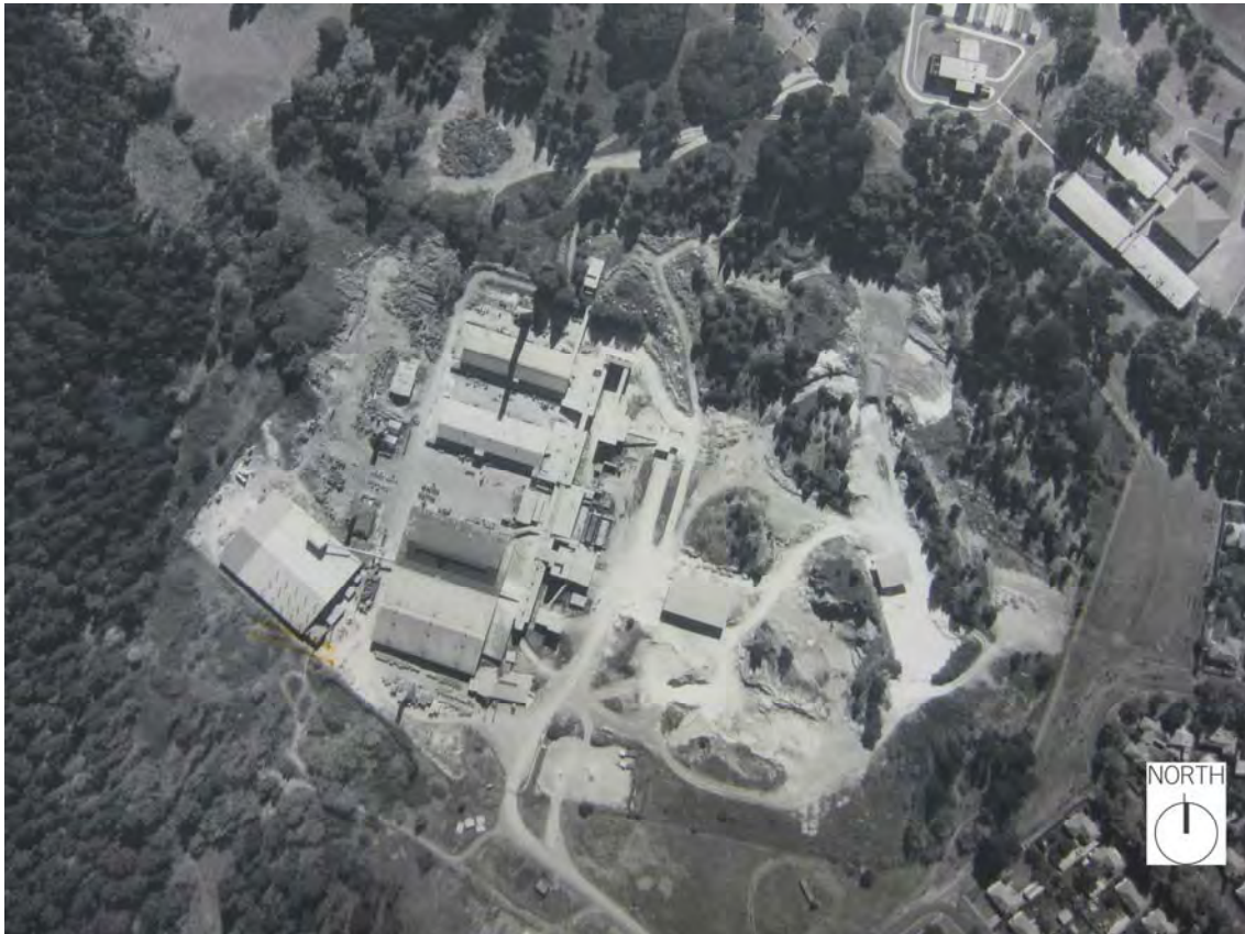
Figure 7 Aerial view, c.1976, at the time of the closure of the Canberra works. At this date, the raw materials had for many years been brought onto the site but the process continued to occur moving from east to west across the site. The 'spine' of process buildings (grinding, crushing, pressing) was located east of the kilns (between the kilns and the quarry).
