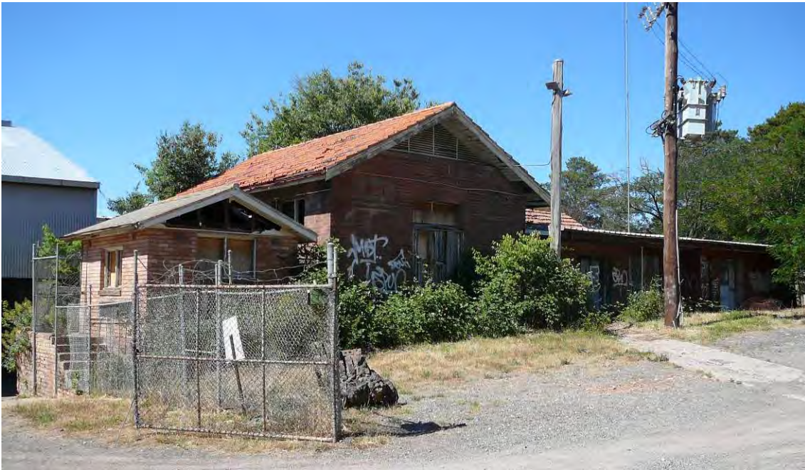
Figure 47 The Power House is the tile roofed building in the centre of the image. The office building (Building 7) adjoins it to the right and the small cream brick structure is the Downdraught kiln control room (Building 23).
