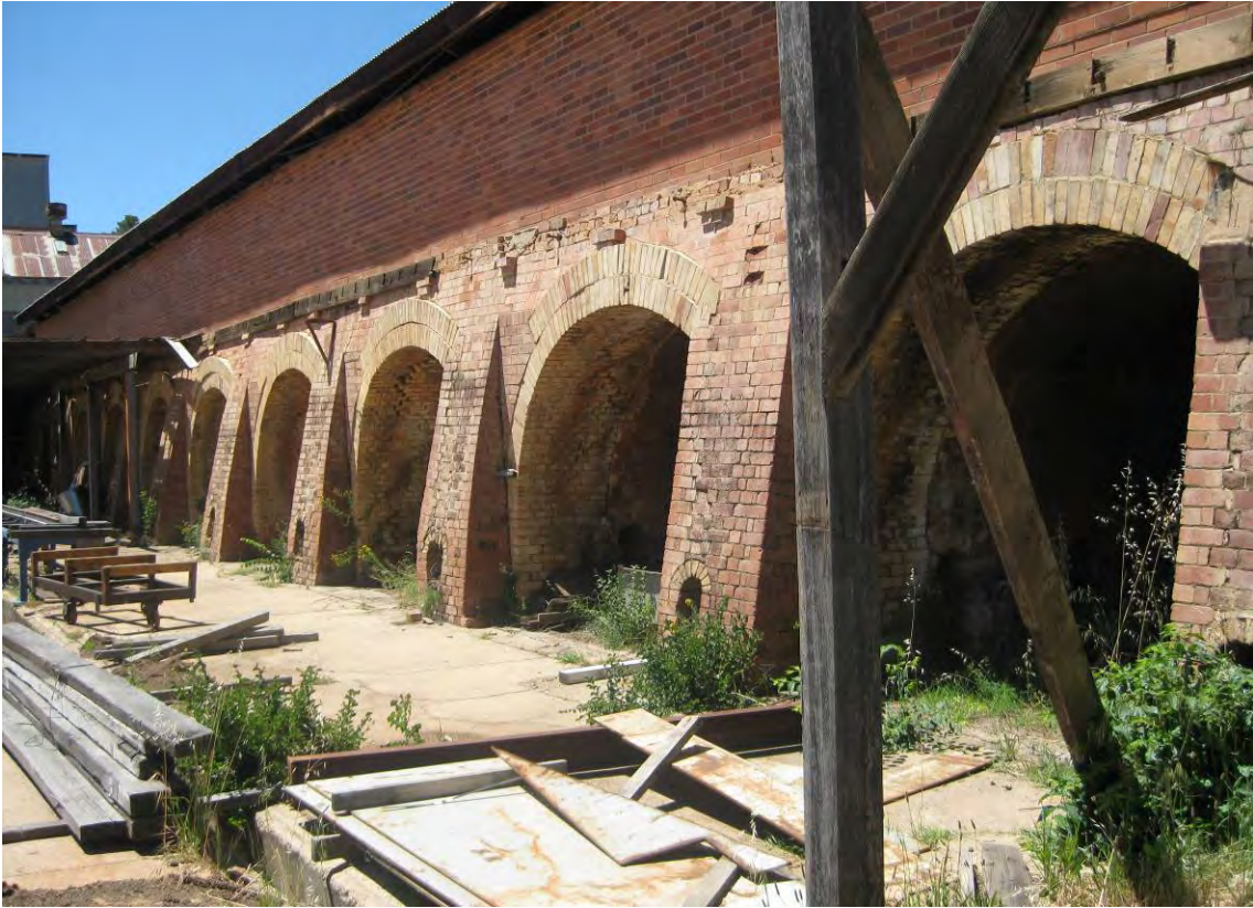
Figure 54 North elevation showing modified kiln entrances.
