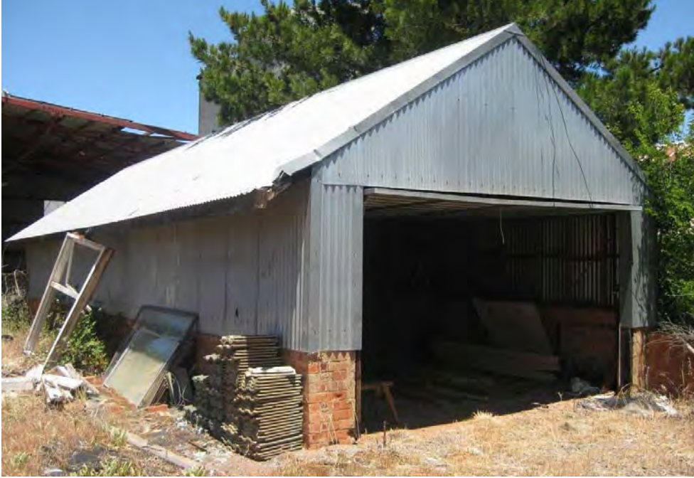
Figure 159 Exterior, showing east and north elevations.
