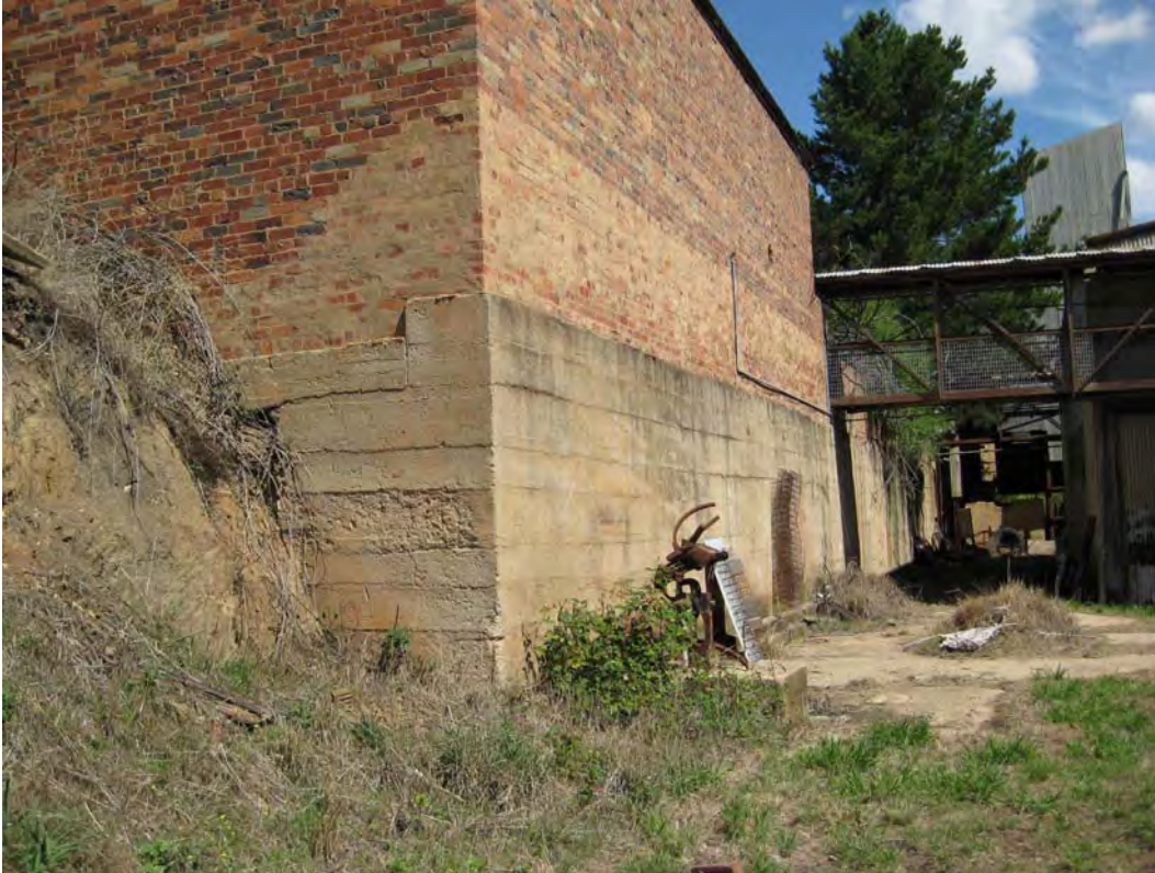
Figure 46 The north end of the concrete wall.
