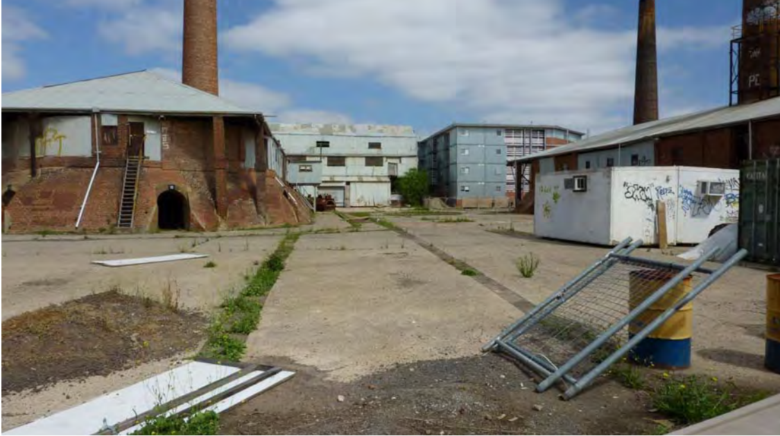
Figure 179 Former Hoffman works at Brunswick, pictured January 2010. Source: Lovell Chen.
