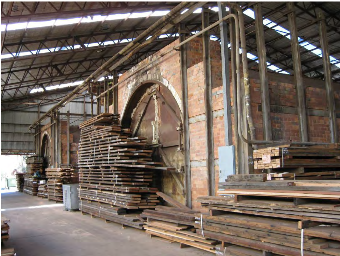
Figure 14 Downdraught kilns numbers 3 and 4 at Canberra Brickworks (Building 22).
