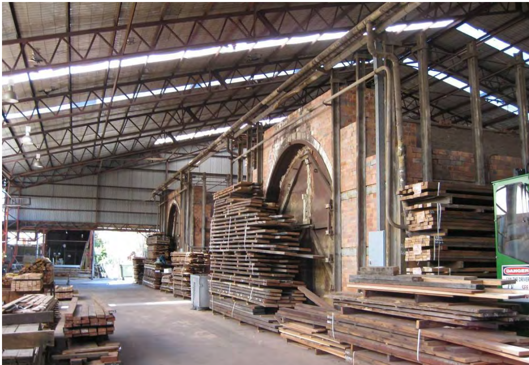
Figure 135 Interior of enclosure showing the north elevation of two of the three kilns.
