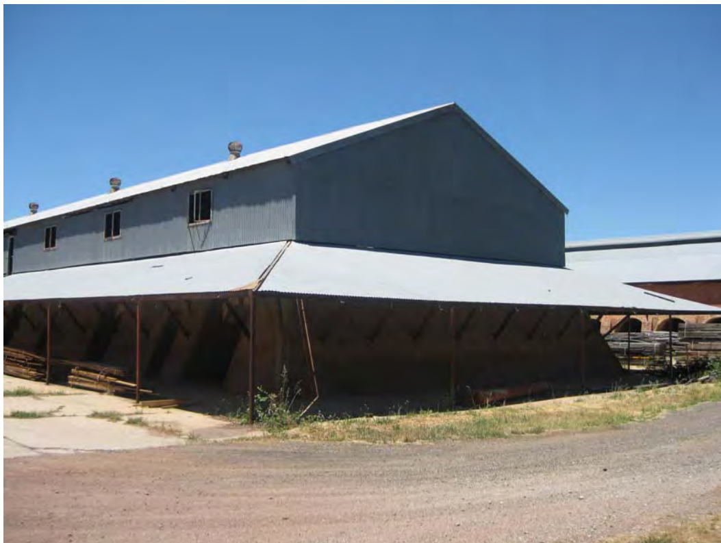
Figure 20 Hardy patent kiln, Canberra brickworks
