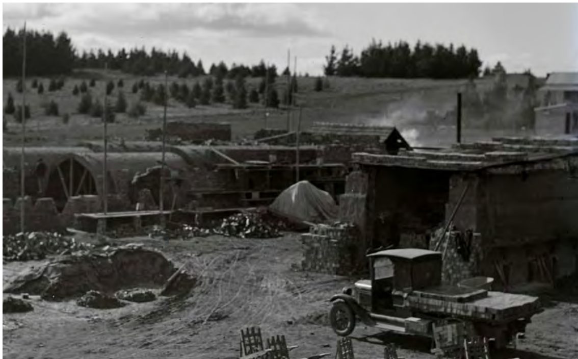
Figure 12 Scotch kiln at Canberra (right), 1926. The first Hardy patent kiln is under construction at the rear of the picture. Source: National Archives of Australia.
