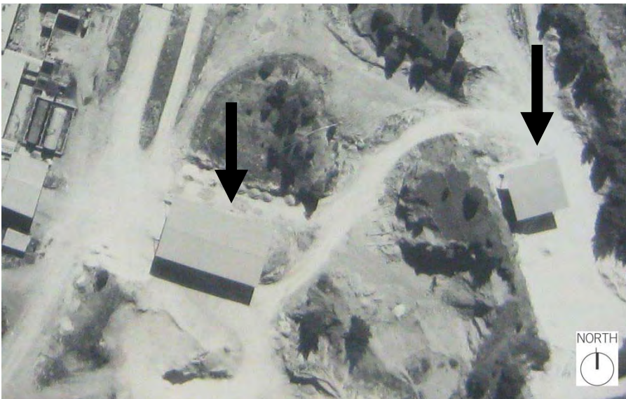
Figure 38 Detail of a 1976 aerial photograph showing the clay storage shed and an unknown smaller structure to the right (both demolished).
