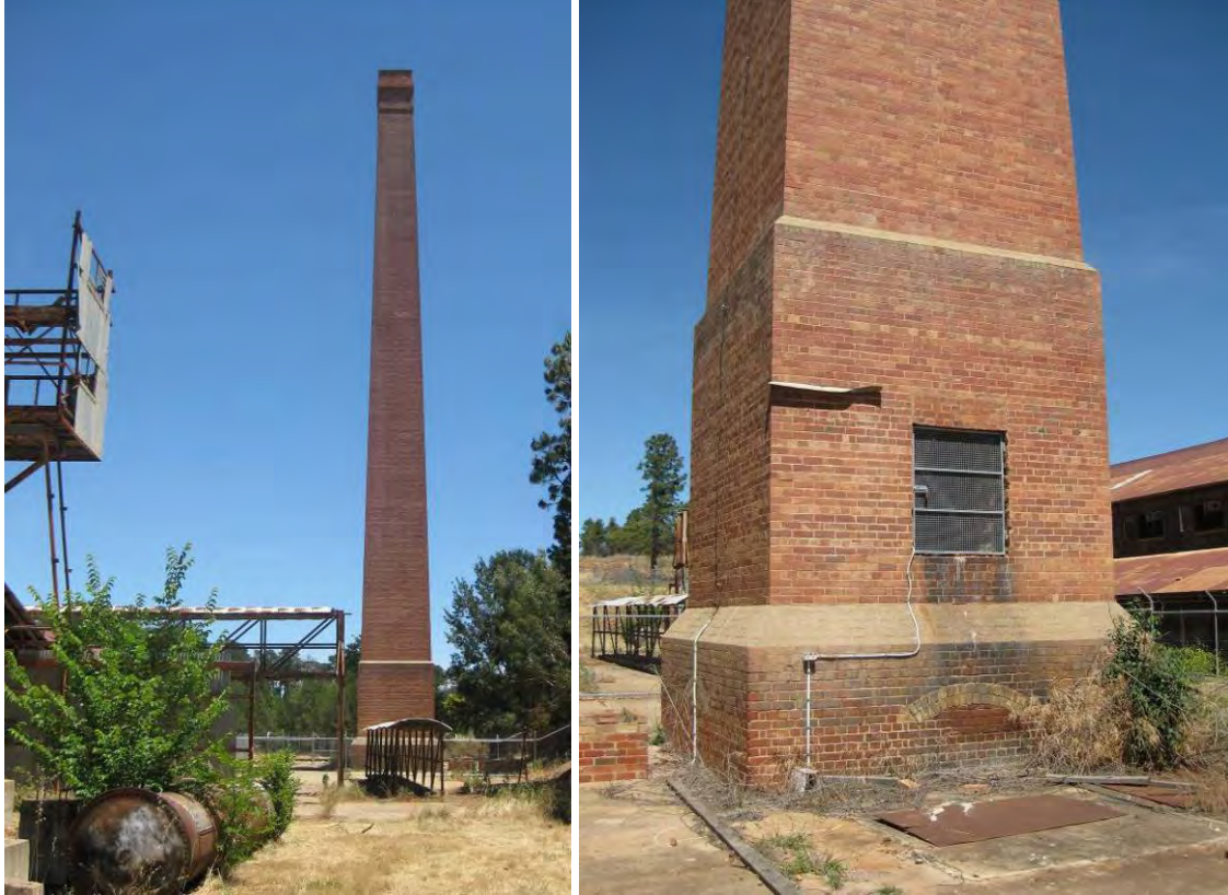
Figure 104 Left: view from east. Right: West elevation, base of stack.
