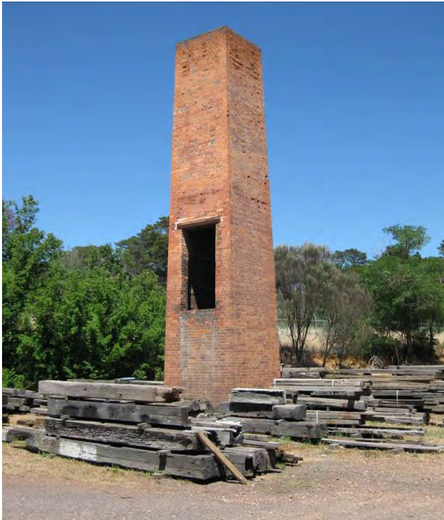
Figure 141 Chimney stack viewed from the north-west.
