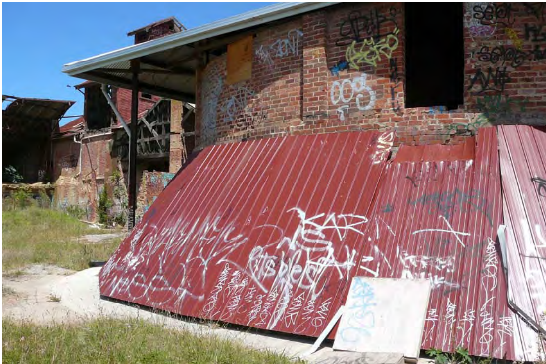
Figure 181 Hoffman kiln at the former Standard Brickworks, pictured in January 2010. Source: Lovell Chen.
