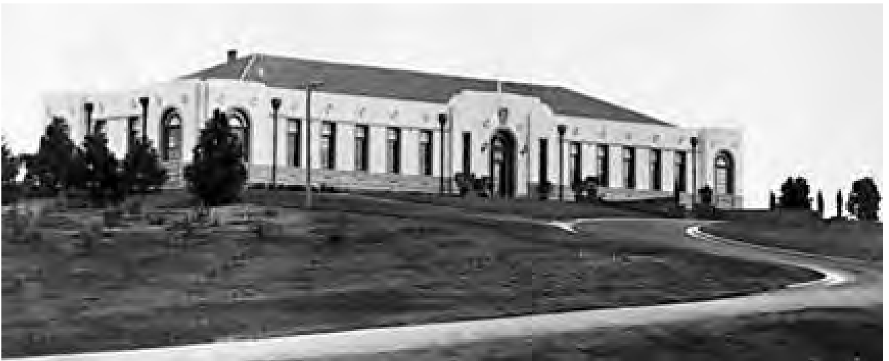
Figure 67 Forestry School, Banks Street, Yarralumla, built 1927.
