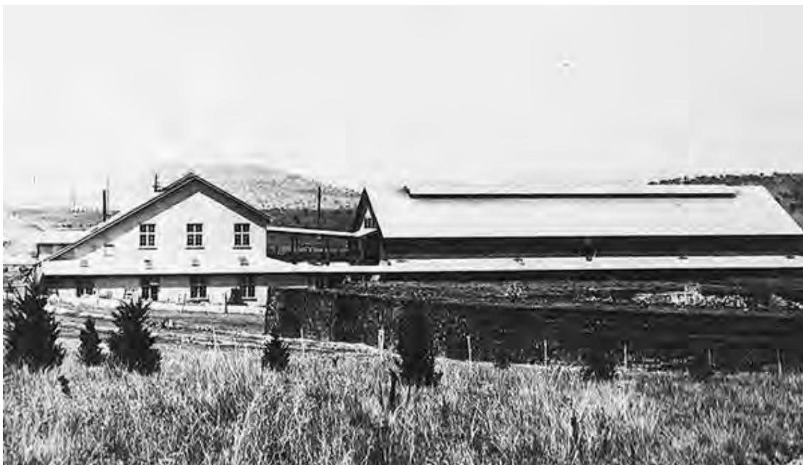
Figure 74 The Machine Shop (left), pictured mid-1920s. Source: National Library of Australia.
