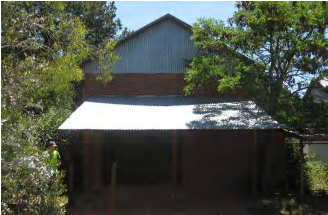
Figure 146 Former boiler house building showing east entry and later verandah addition.
