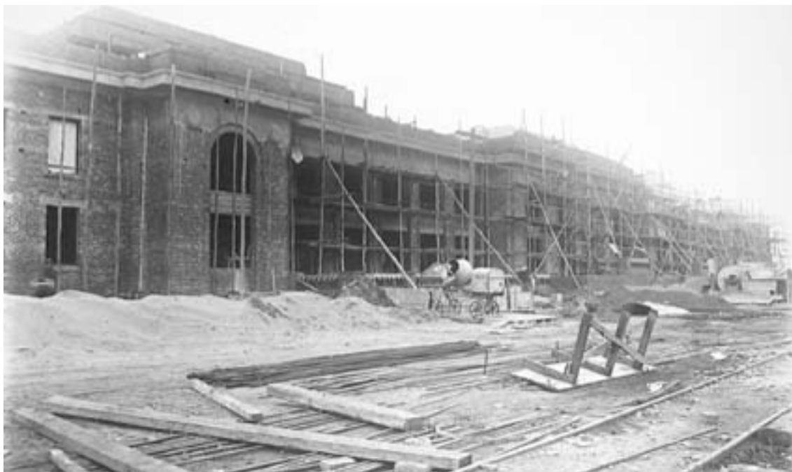
Figure 187 Parliament House prior to rendering (1926), with brickworks railway in foreground.
