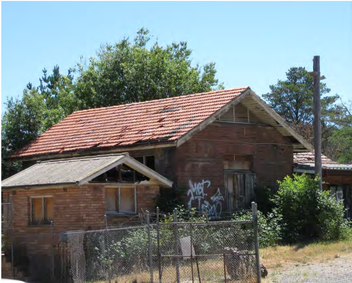
Figure 140 The downdraught kiln control room is the cream brick building adjoining the larger terracotta-tiled Power House (Building 3).
