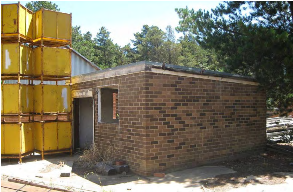
Figure 148 The storage building, adjoining the site of the brick extrusion plant site.
