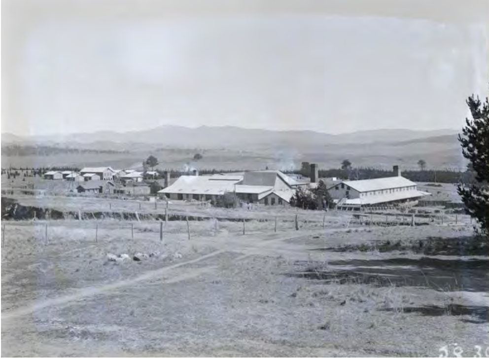
Figure 196 View west of the complex in 1929, including part of the quarry, the kilns and their stacks (albeit the Staffordshire kiln obscured), and the office and Power House (on left). The original crushing and pressing buildings (now demolished) are in the centre of this view, to the left of the Hardy patent kiln and in the background (far left) is the Brickworks Camp complex, now demolished. Source: National Library of Australia.
