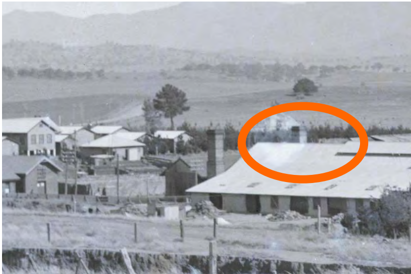
Figure 134 Detail from a 1929 photograph of the brickworks, with the chimney of the temporary downdraught kilns highlighted. Source: National Archives of Australia.
