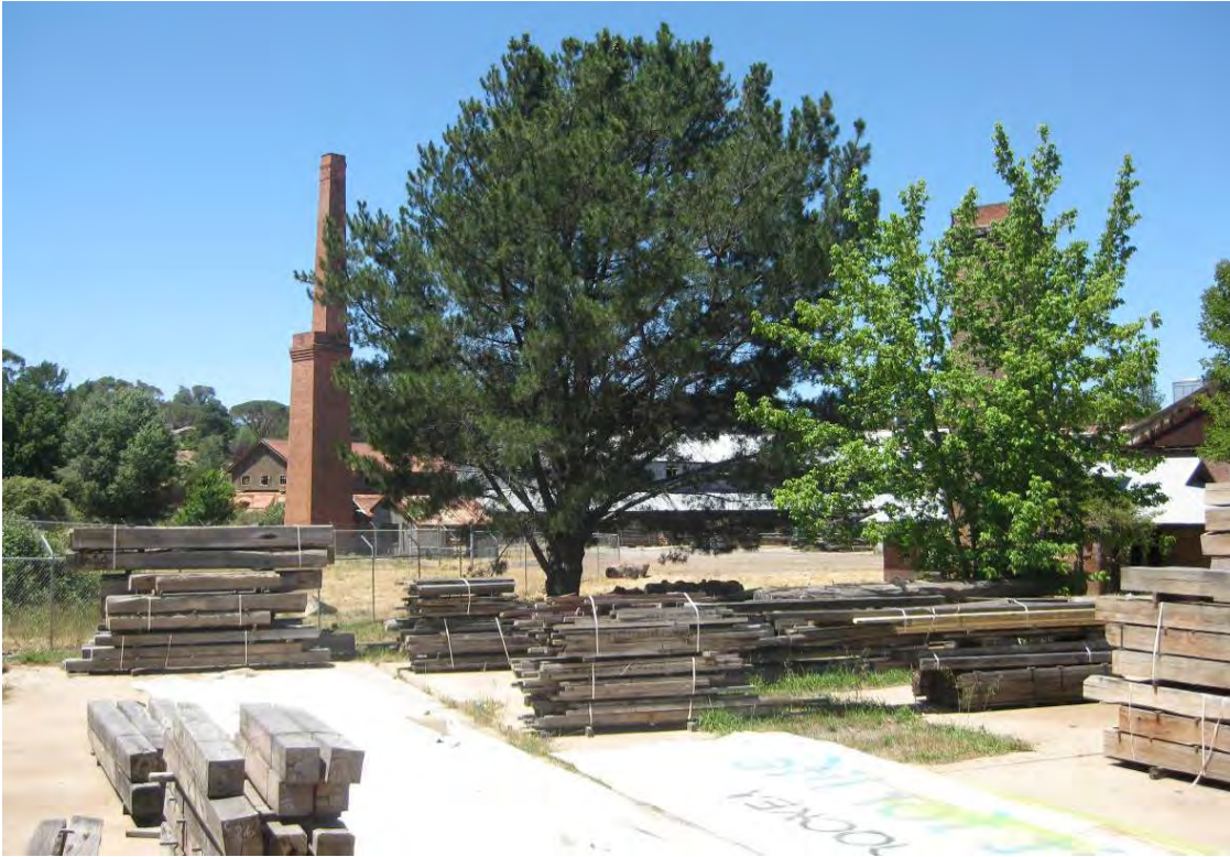
Figure 150 Brick extrusion plant site, looking north-east.
