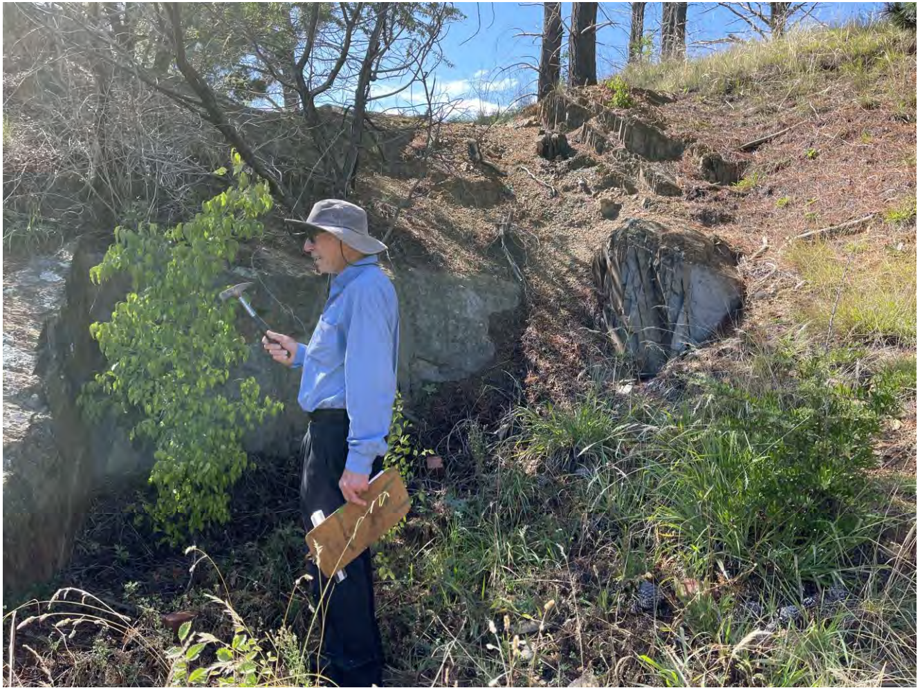
Photo 9 – 22/2/2021 – View of Location 8A, showing the rock face to comprise foliated, MW/SW Phyllitic Mudstone.
