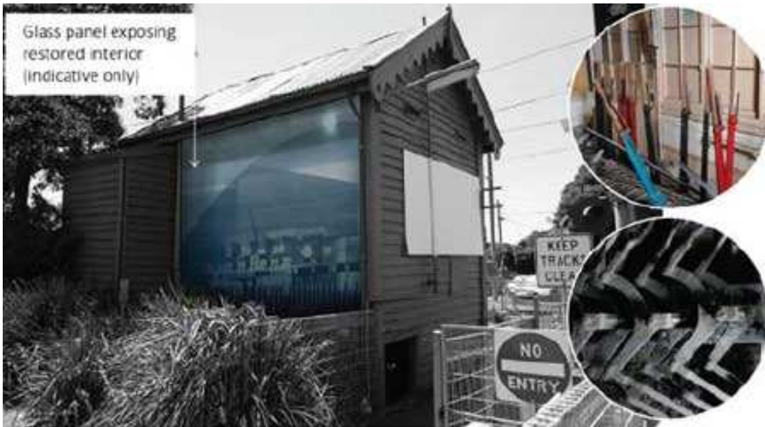
Figure 10 Proposal for partial removal of timber wall to a signal box to ‘reveal’ the intact gears and mechanisms within
