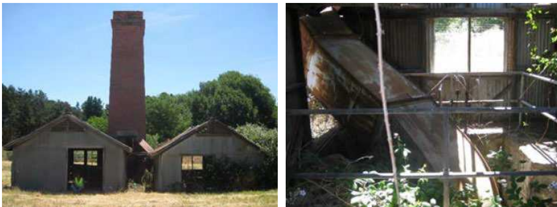
Figure 9 Left: Hardy Patent kiln 1, exterior; Right: Hardy Patent kiln 1, interior
