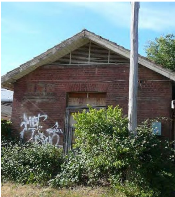
Figure 3 South elevation and entry, showing bricked up openings. (Source: Lovell Chen, 2010, Canberra Brickworks CMP, p 56)
