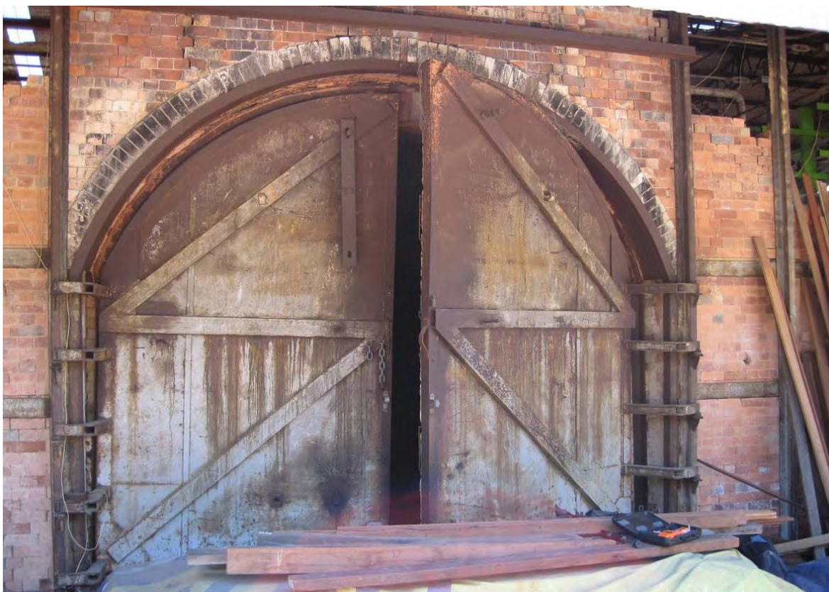
Figure 5 Kiln entry showing stepped side wall. (Source: Lovell Chen, 2010)
