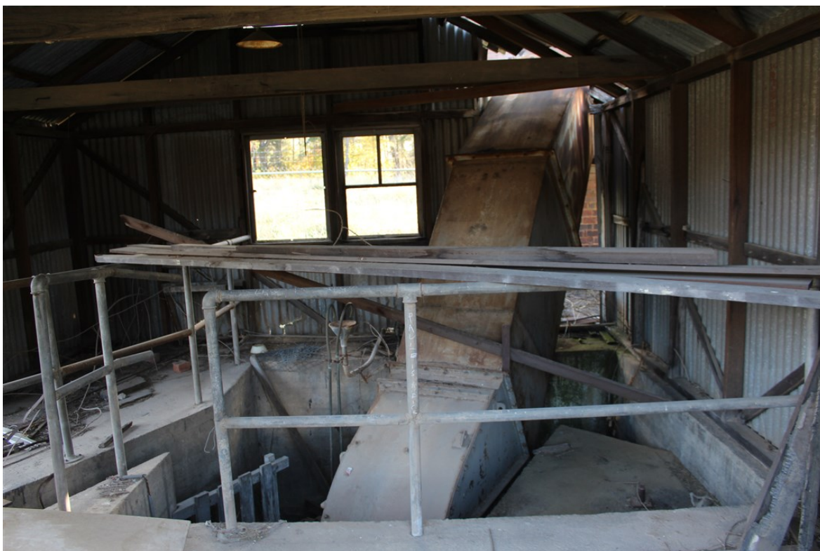
Figure 3 Interior of the c1955 structure showing the duct leading to the chimney stack. (Source: GML, 2017)
