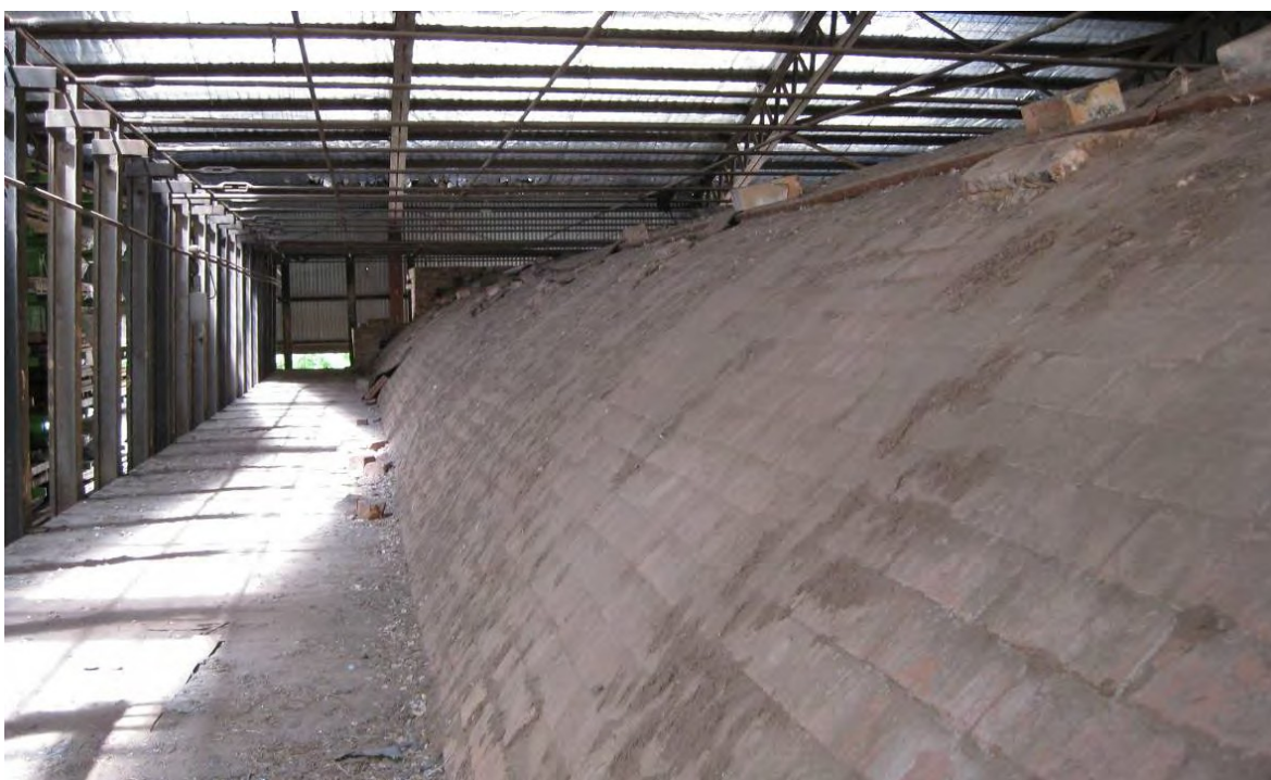
Figure 4 Kiln roof with brick walkway to sides. (Source: Lovell Chen, 2010)
