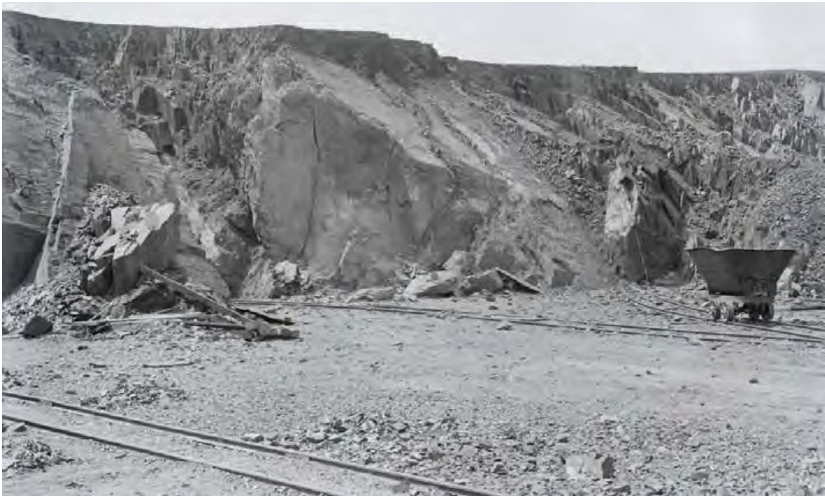
Figure 1 View of the quarry showing the narrow-gauge tramway used to transport shale to the crusher, 1921. (Source: National Archives of Australia)
