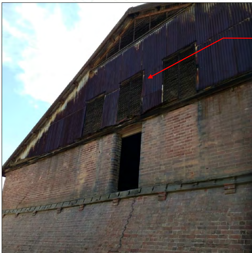
Deteriorated wall sheeting
