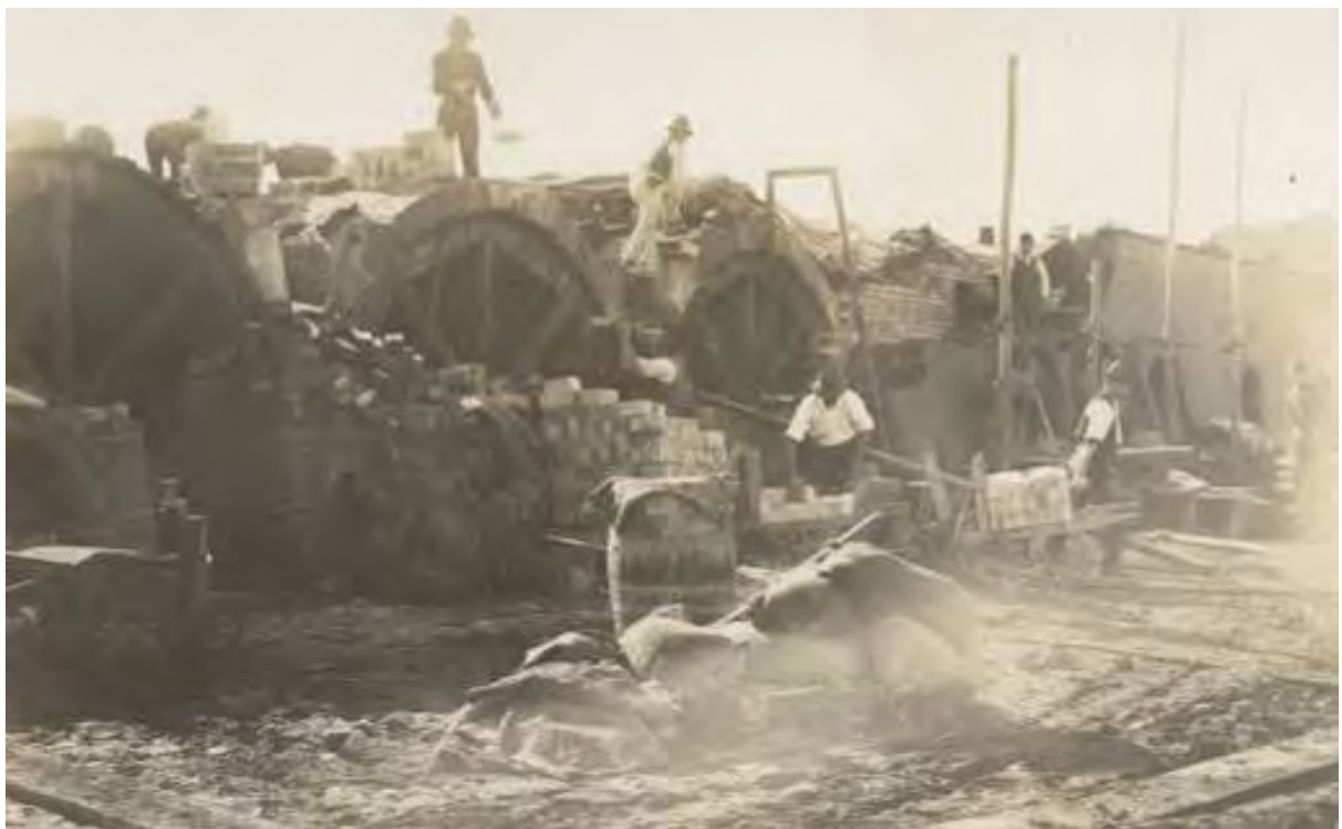
Figure 29 Constructing the transverse arches of the Staffordshire Kiln, c1915. (Source: National Library of Australia)
