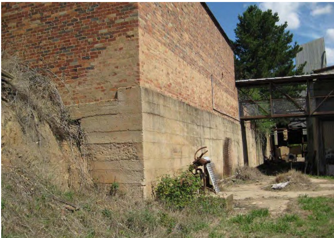
Figure 3 The north end of the concrete / brick retaining wall. (Source: Lovell Chen, 2010)
