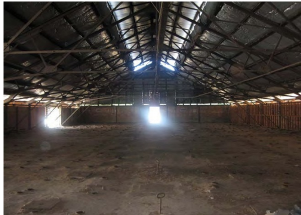
Figure 19 Interior of the firing floor to one of the Hardy patent kilns at the Brickworks. (Source: Lovell Chen, 2010, Canberra Brickworks CMP, p 30)
