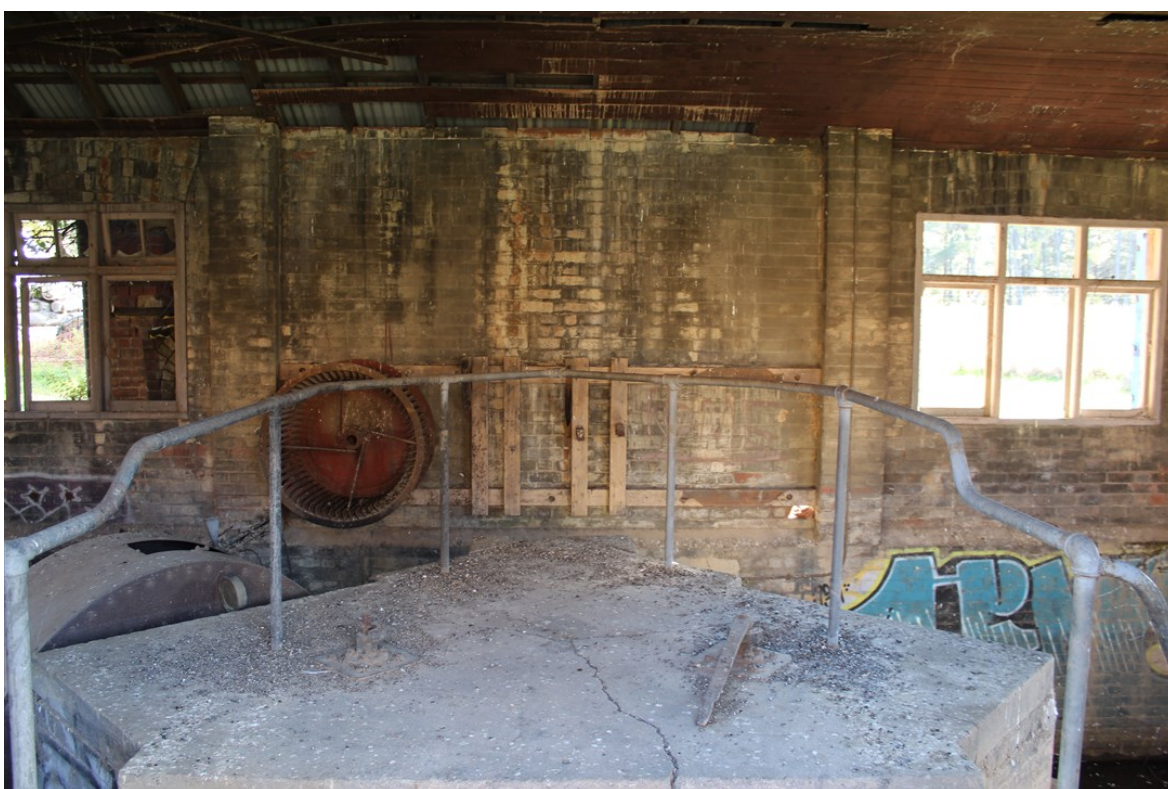
Figure 3 Interior of the Fan House from entrance across ground level platform. Tangential fan mounted on rear wall. (Source: GML, 2017)
