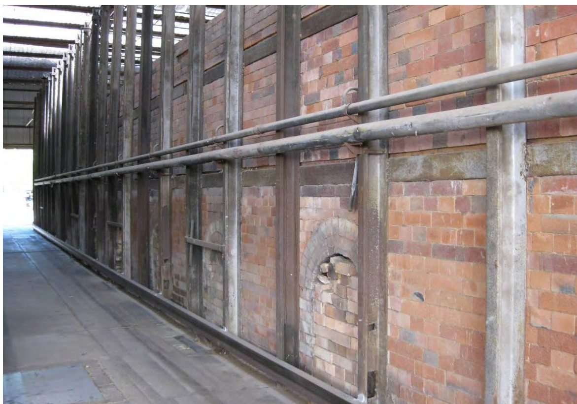
Figure 6 Side elevation showing steel framing and fire holes. (Source: Lovell Chen, 2010)
