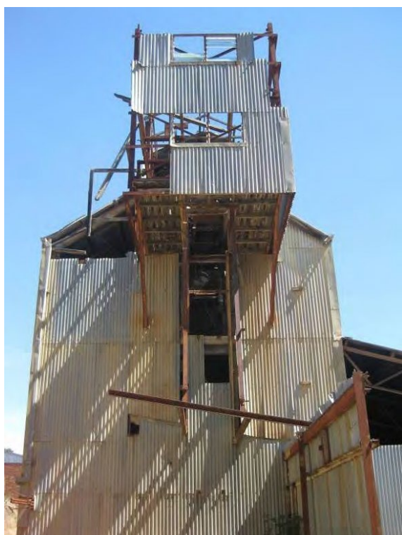
Figure 6 North end of Machine Bay 3 showing remains of headgear housing for the loft conveyor. (Source: Lovell Chen, 2010)
