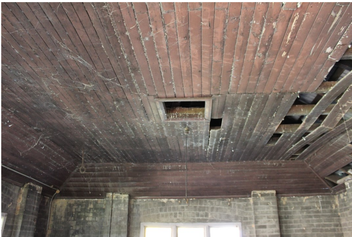
Figure 4 Interior of the Fan House, showing poor condition ceiling boards. (Source: GML, 2017)
