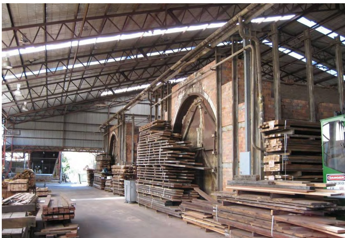
Figure 3 Interior of enclosure showing the north elevation of two of the three kilns, under the large steel roof, a later addition. (Source: Lovell Chen, 2010)
