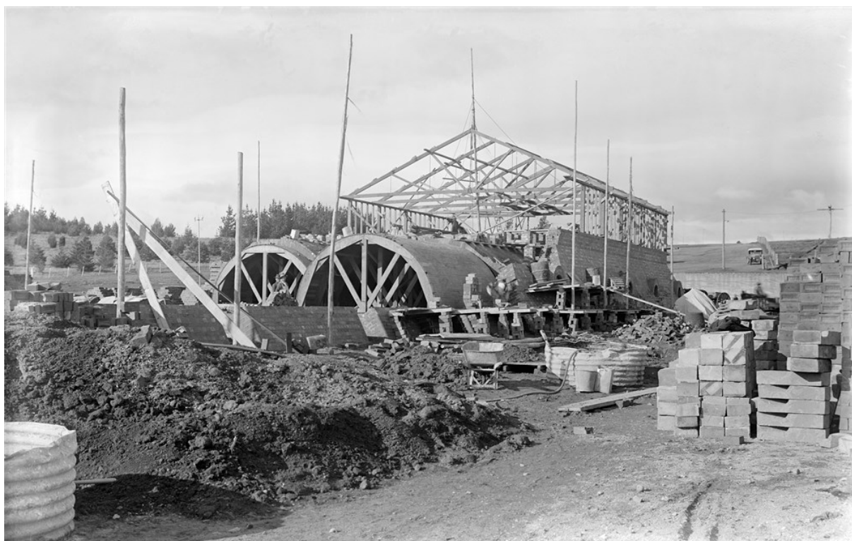
Figure 43 Hardy Patent Kiln 1 under construction, c1926. (Source: National Archives of Australia)
