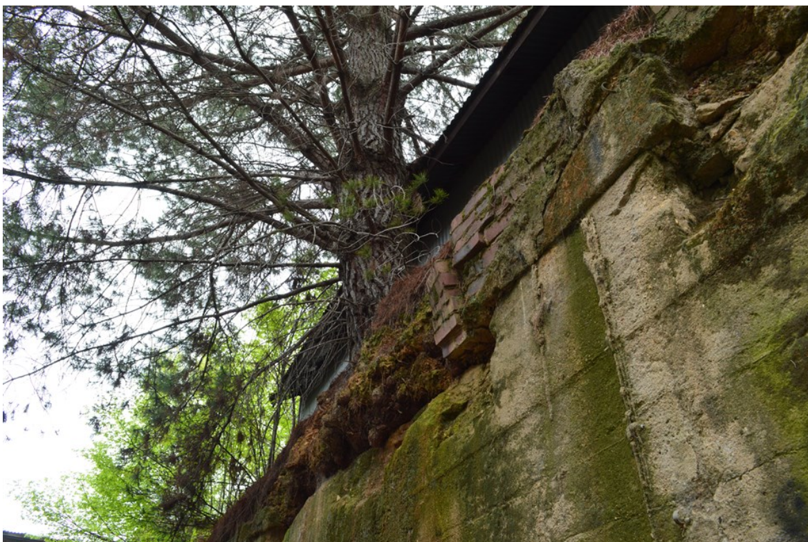
Figure 4 Top of retaining wall showing unstable tree. (Source: GML, 2016)
