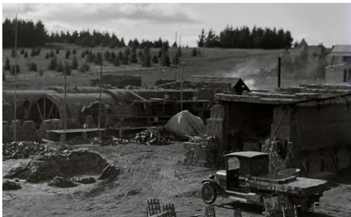
Figure 9 Scotch kiln at the Brickworks (right), 1926. The first Hardy patent kiln is under construction at the rear of the picture. (Source: National Archives of Australia)
