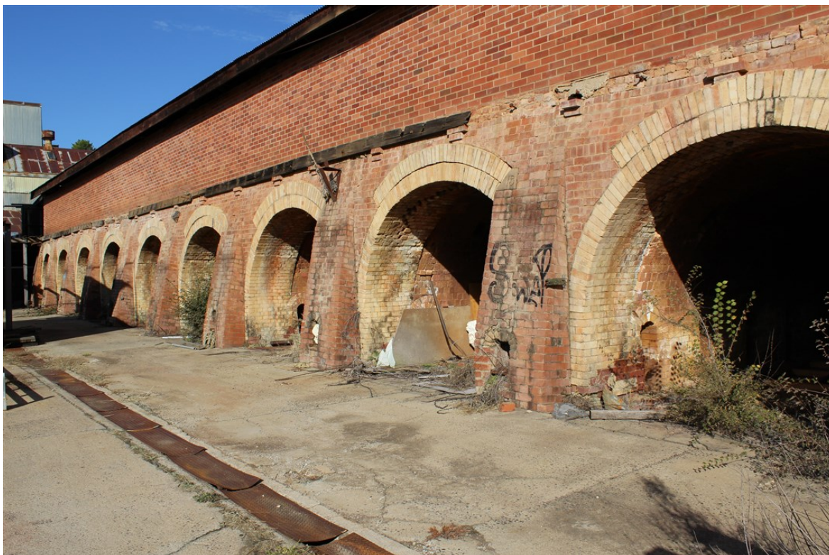
Figure 7 North elevation showing modified kiln entrances. (Source: GML, 2017)
