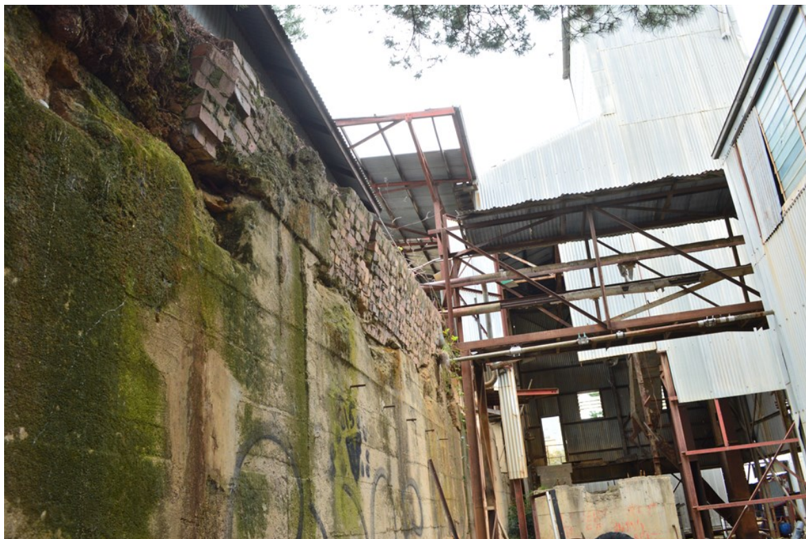
Figure 5 Concrete top and upper masonry work to the retaining wall partially collapsed. (Source: GML, 2016)
