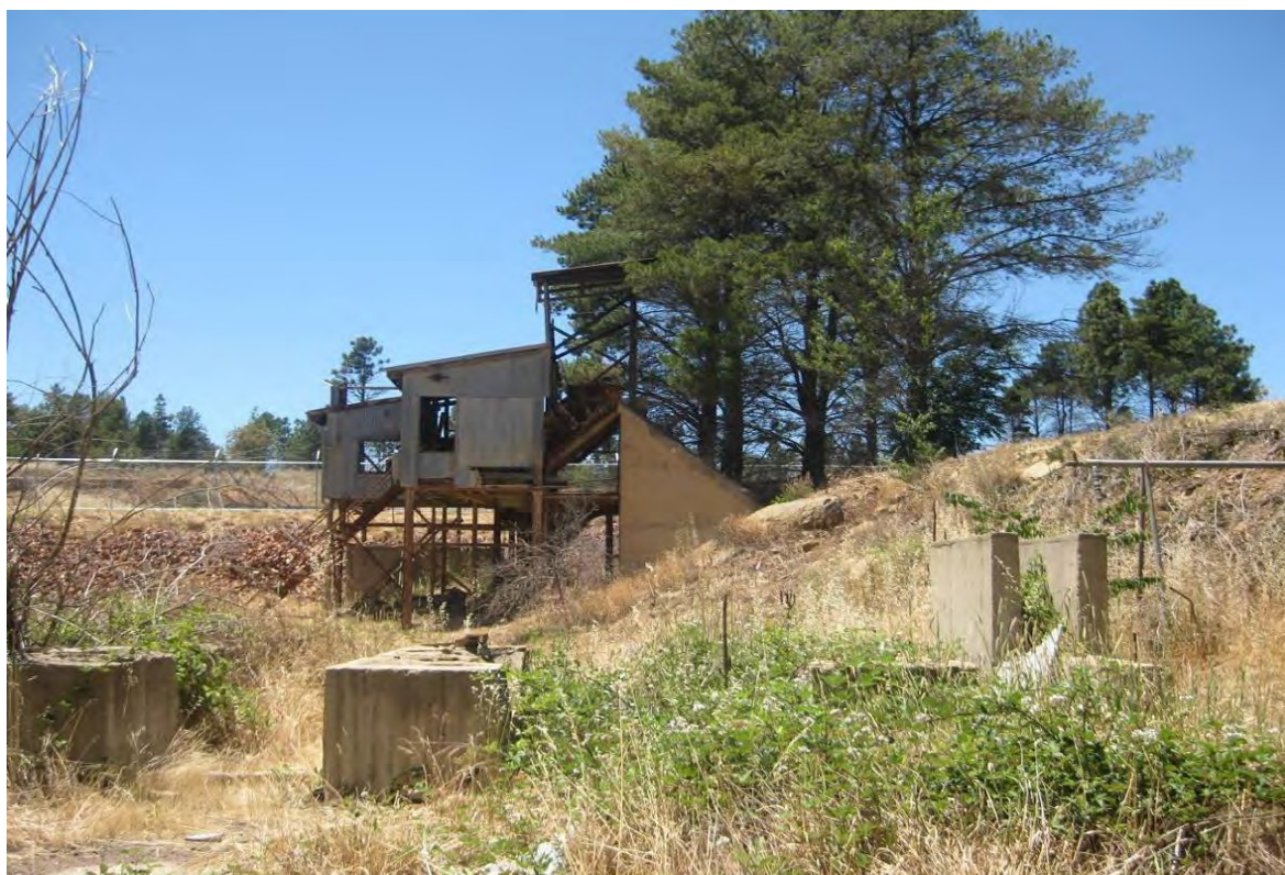
Figure 4 The Primary Crusher House viewed from the west. The concrete footings in the foreground supported the now demolished conveyor which transported crushed material to the Red Pan Room (also demolished) for further refining. (Source: Lovell Chen, 2010)
