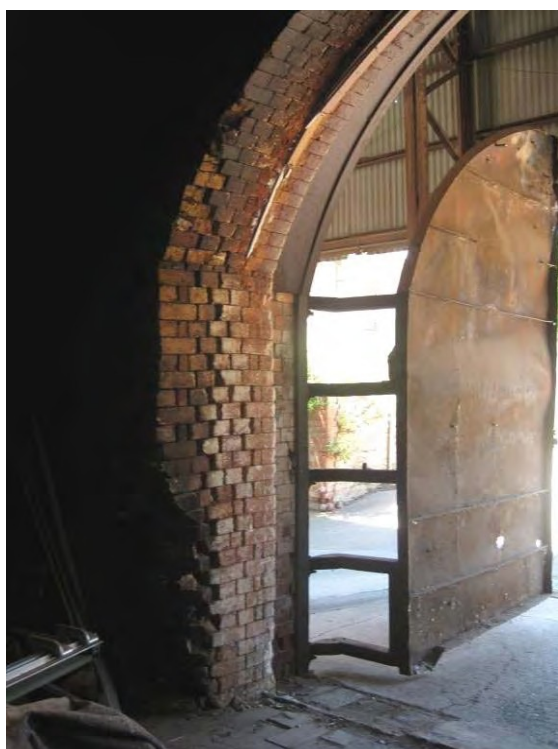
Figure 7 Interior of kiln showing entry and deteriorating fire bricks. (Source: Lovell Chen, 2010)
