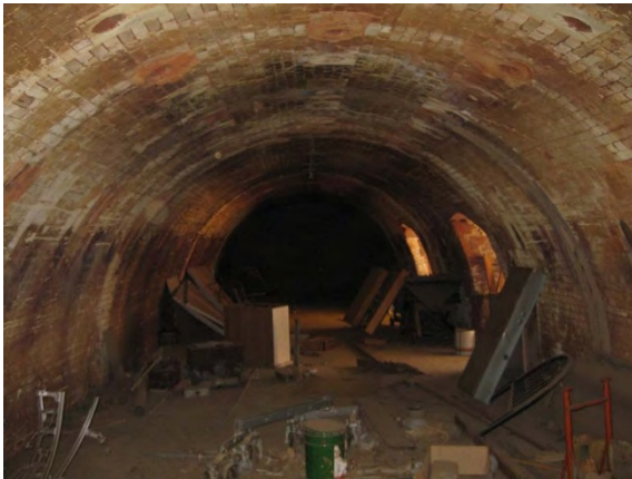
Figure 18 View into the firing chamber of one of the Hardy patent kilns at the Brickworks. Note the wickets (openings) on the right where the bricks were loaded and unloaded, and the firing holes in the ceiling/walls. (Source: Lovell Chen, 2010, Canberra Brickworks CMP, p 30)
