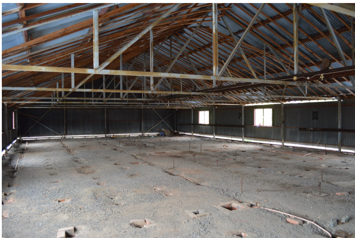
Figure 6 First floor of Hardy Patent Kiln 1 with firing holes visible to the floor. (Source: GML, 2017)
