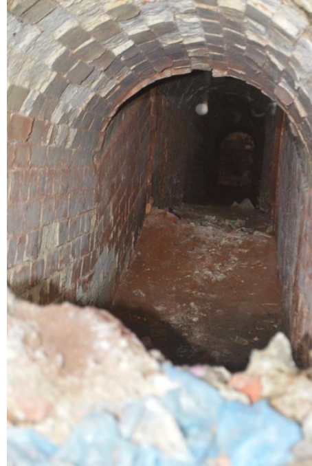
Figure 4.137 Left: the entrance to Tunnel B from the central tunnel. Right: the inclined slope in the north-south portion of Tunnel C, showing the rear wall of the flue where it exits at the northern-most vent adjacent to the northern wicket of the central Downdraught Kiln. Note: the B and C tunnels are mirrored, so these characteristics are present in both tunnels.
