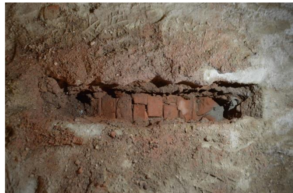
Figure 4.129 An intact brick flue.
