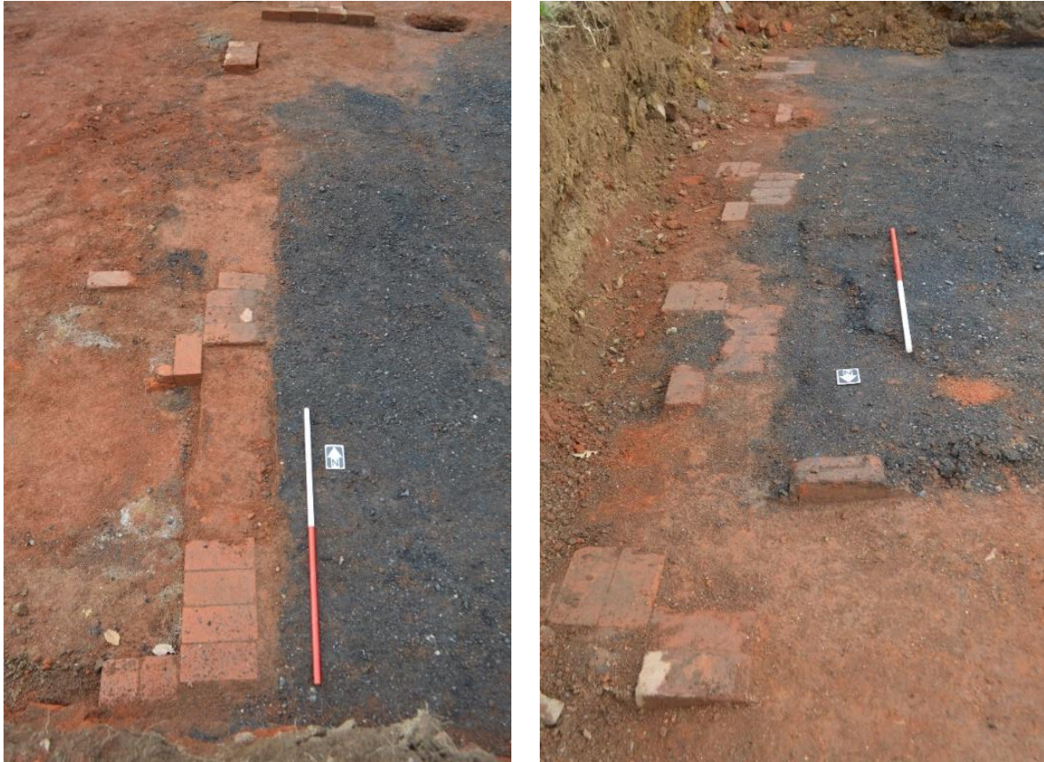
Figure 4.85 OA2, the western (196, left) and eastern (195, right) external walls, facing various.
