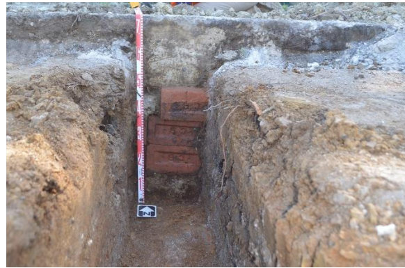
Figure 4.113 TT3, the stack of unbonded bricks (19) abutting the external wall of the sunken footings (18), aspect north.
