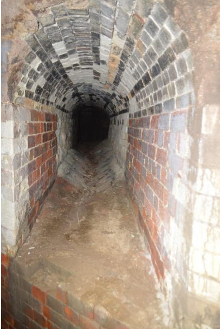
Figure 4.137 Left: the entrance to Tunnel B from the central tunnel. Right: the inclined slope in the north-south portion of Tunnel C, showing the rear wall of the flue where it exits at the northern-most vent adjacent to the northern wicket of the central Downdraught Kiln. Note: the B and C tunnels are mirrored, so these characteristics are present in both tunnels.
