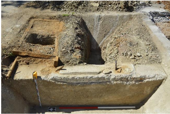
Figure 4.112 TT3, eastern basin of the sunken footings (18) showing the compact clay fills (23 and 24), aspect east.
