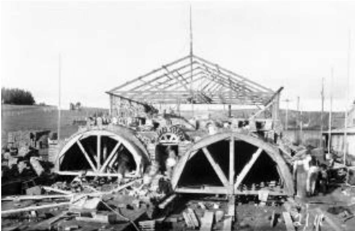
Figure 2.7 The Hardy Patent Kiln 1 under construction, c1926. (Source: NAA, A3560 2111)
