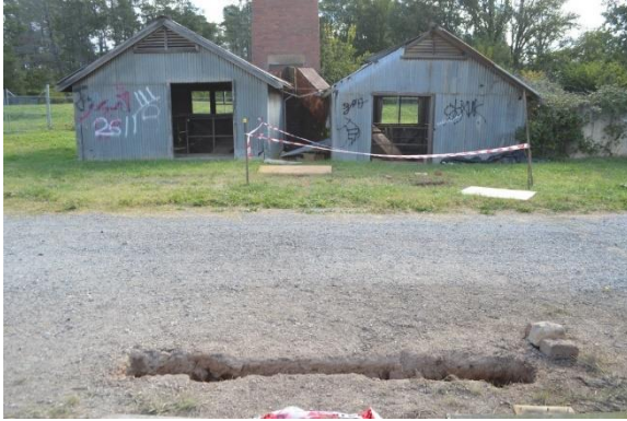
Figure 4.125 GPR identified a single tunnel leading from the fan houses to the kiln, which enters the kiln at the location of the 'Kent' oxygen analyser.
