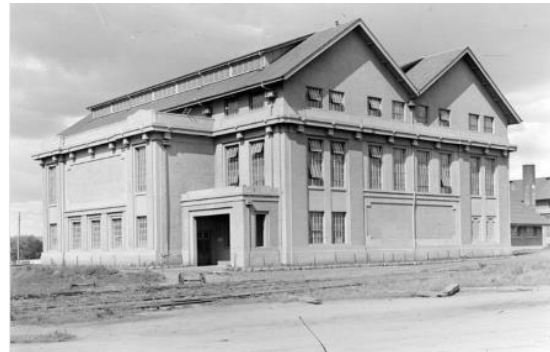
Figure 2.2 The Kingston Powerhouse, c1926. (Source: NAA, A3560 150)
