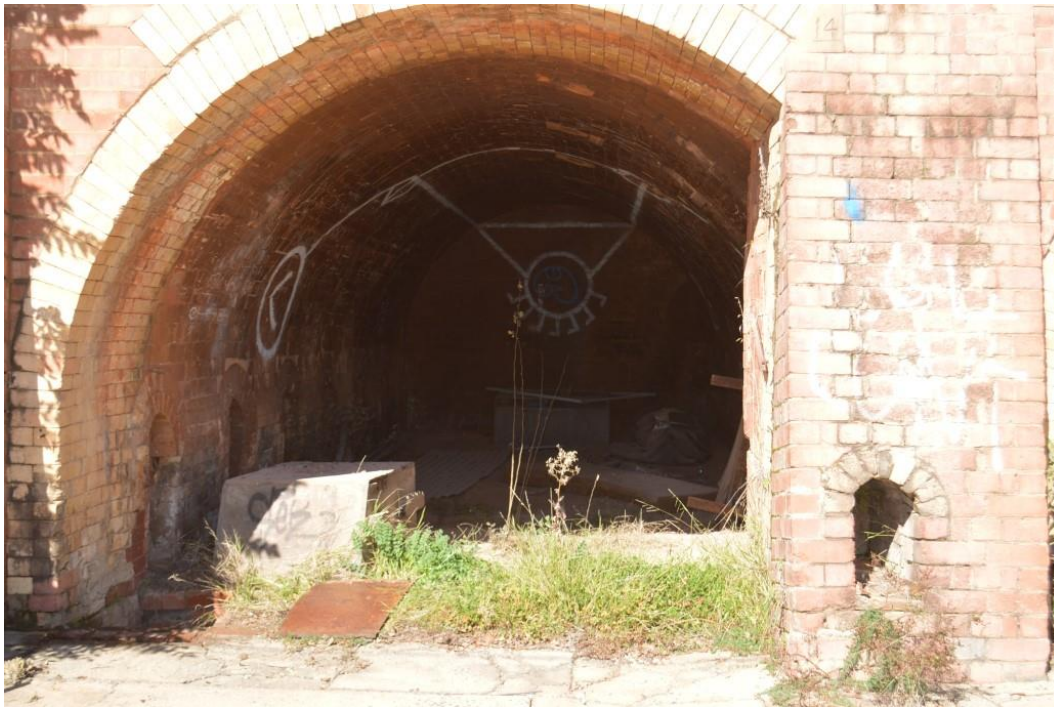
Figure 4.121 Each smaller flue channel leads to an individual kiln chamber, where it meets the surface in two locations—one in the floor surface within the wicket (front left, visible adjacent to internal wall) and one in the external wall adjacent to the wicket (right, visible as arched opening).
