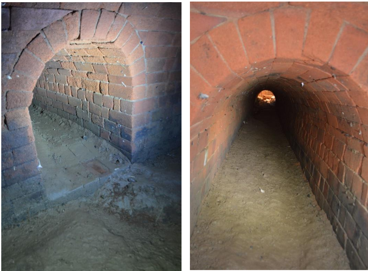
Figure 4.120 One of the smaller flue channels leading off the central tunnel.
