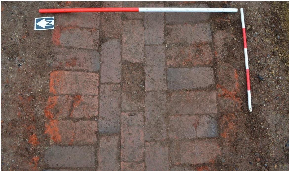
Figure 4.42 OA1, the spoon drain (50), facing east. The drain was constructed from three stretcher rows, guttered by a single row of soldiers. An additional stretcher row capped the soldiers in some places (right).
