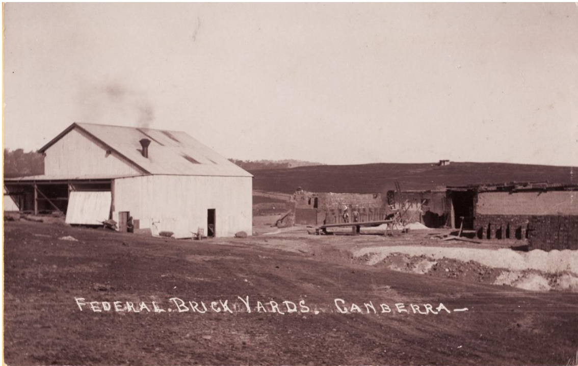
Figure 4.101 Photograph of the experimental plant. This photograph was taken from the same angle as Figure 4.100, but likely shows an earlier stage of the experimental plant. (Source: CDHS, 2295).
