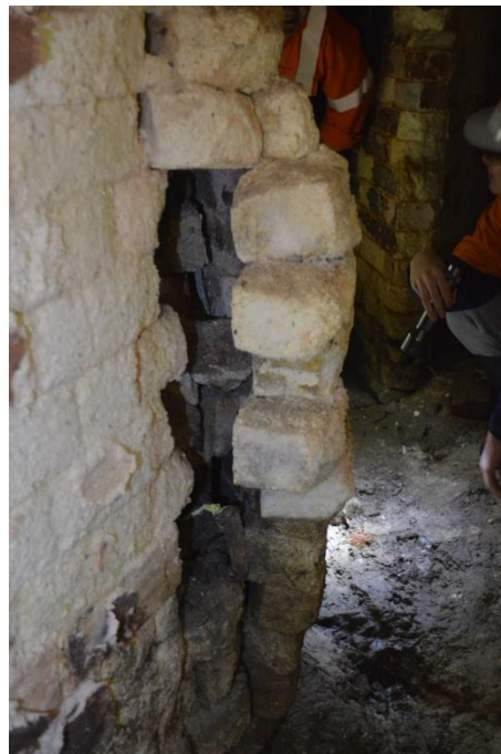
Figure 4.141 Damp conditions have resulted in extensive salt damage and cracking in the brickwork (see also Figure 4.136).
