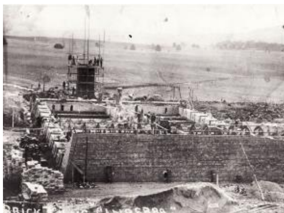
Figure 2.3 Staffordshire Kiln construction at the Brickworks, c1915. (Source: Canberra District Historical Society, ID15652)
