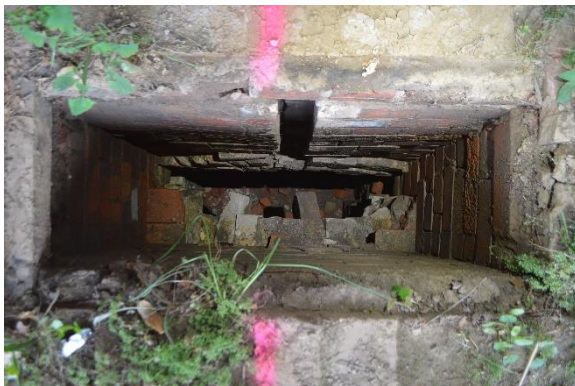
Figure 4.139 Top: western side of the western Downdraught Kiln, showing the southern vent aligned with the wicket. Bottom left: view down the southern vent aligned to the eastern side of the western Downdraught Kiln. Bottom right: northern vent aligned to the western side of the eastern Downdraught Kiln.
