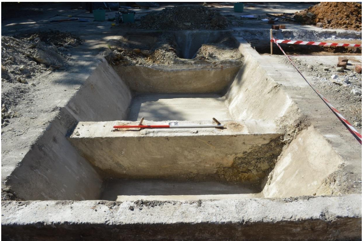
Figure 4.111 TT3, the sunken footings (18), aspect east.
