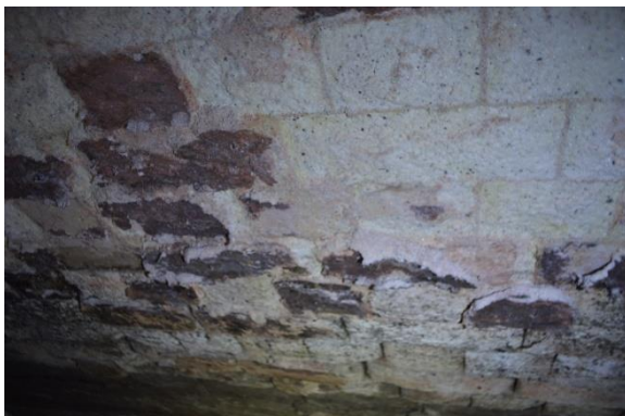
Figure 4.141 Damp conditions have resulted in extensive salt damage and cracking in the brickwork (see also Figure 4.136).
