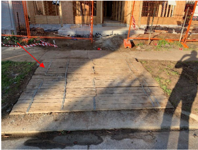
Figure 3: Example of rumble boards used for ground protection. If used for vehicular traffic, boards must be installed over 200mm of coarse mulch.
