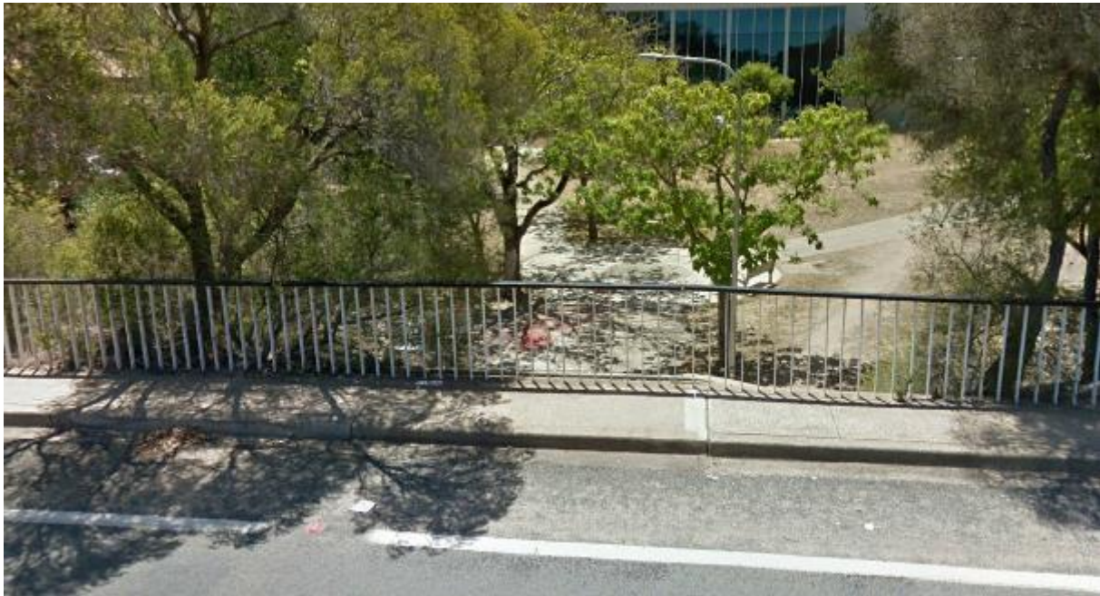
Figure 16 Narrow footpath on Melrose Drive at underpass
