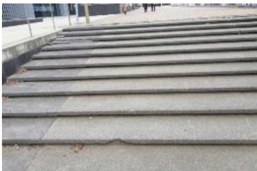
Figure 20 Furzer Street and Westfield link
