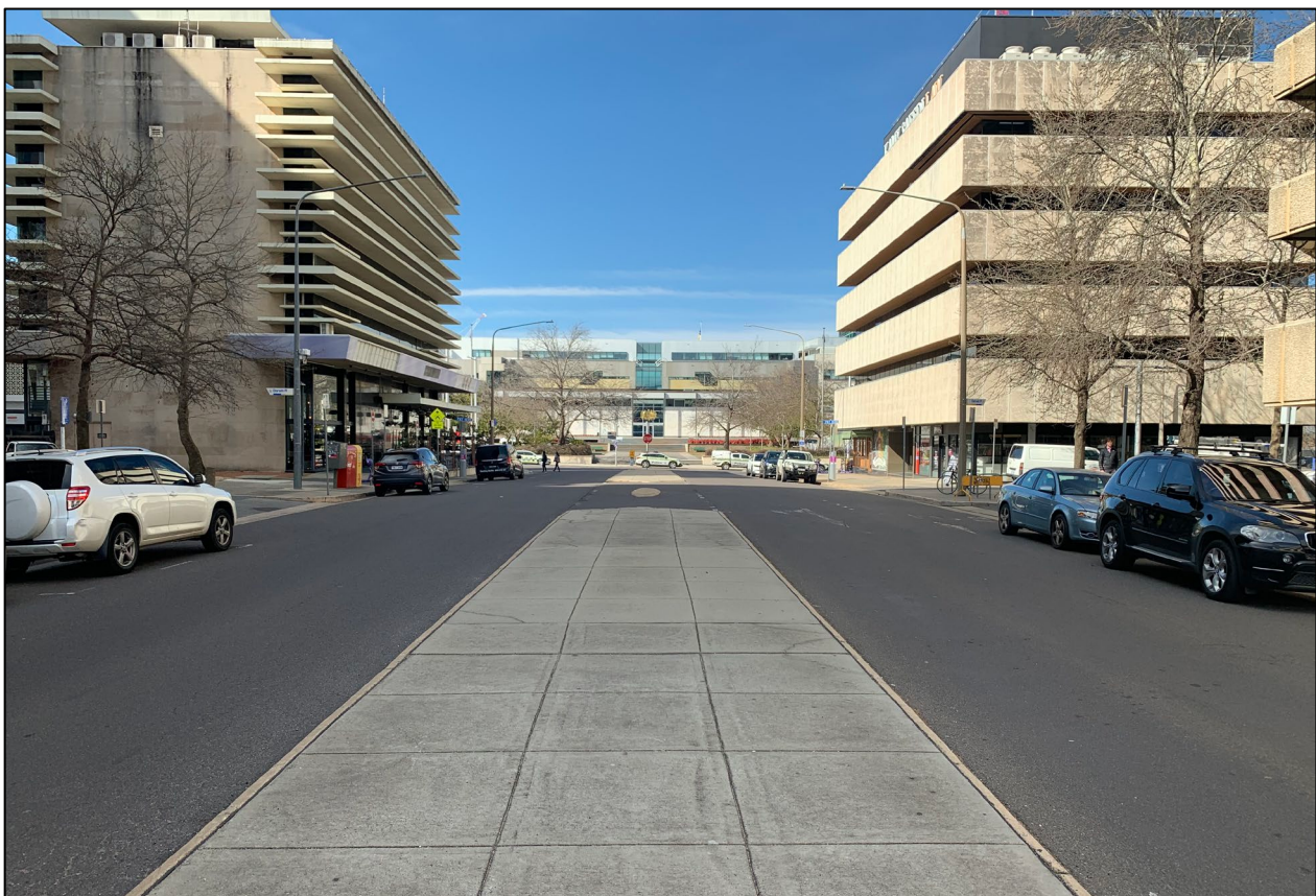
Figure 4 University Avenue, looking southeast towards break in median opposite Darwin Place
