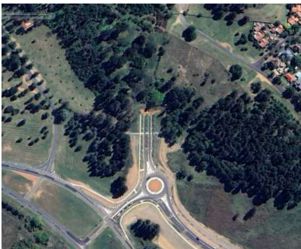
Southern extent of Block 7 Google Earth Image March 2022
