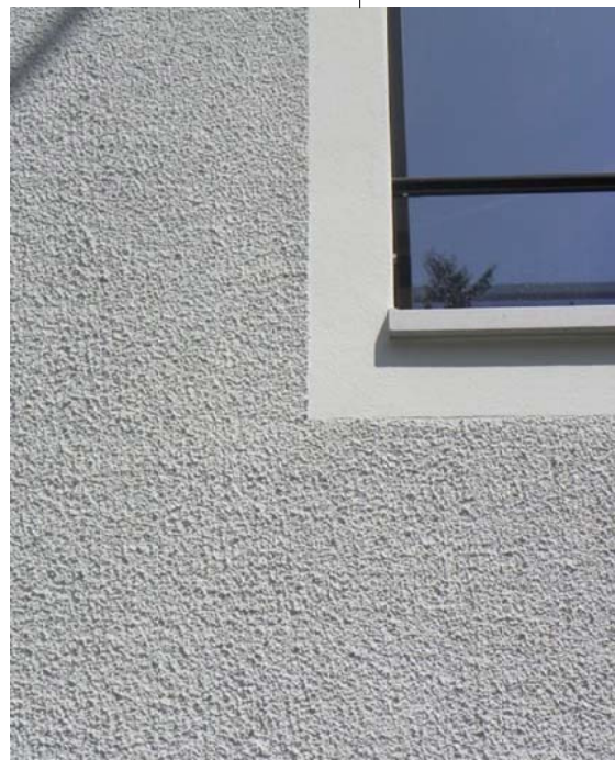
TYPICAL WALL FINISH HEAVY TEXTURED RENDER (TERRALINE) PAINTED OFF WHITE
