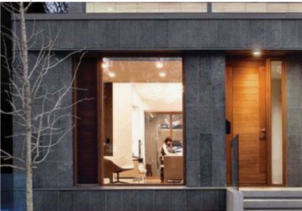
STONE SPANDREL FINISH BLUESTONE / BASALT VENEER BETWEEN WINDOWS LOWER AND UPPER LEVELS
