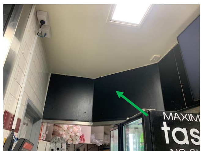
Photograph 6: Internal; Upper wall lining above menu screens containing no asbestos.
